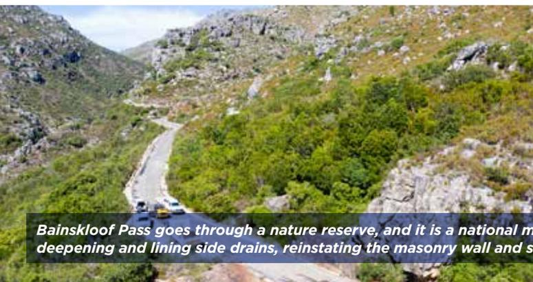
*Bainskloof Pass goes through a nature reserve, and it is a national monument. Work included repairing and resealing the existing road, deepening and lining side drains, reinstating the masonry wall and stone boulders, and stabilising certain slopes.*
