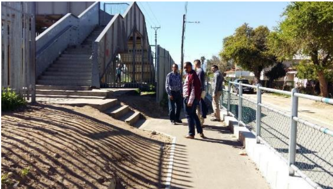
Figure 3-4 Before and after, Klapmuts, Beyers Street access to rail station
