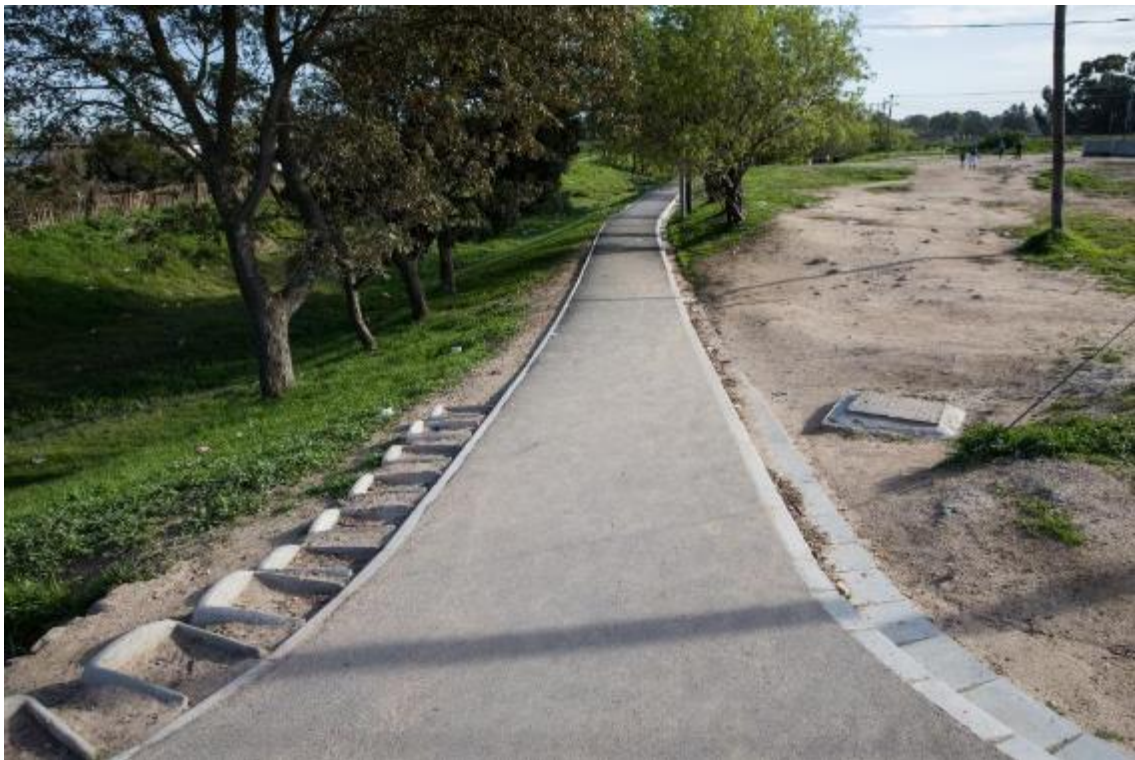
Figure 3-3 Before and After, Klapmuts linking Beyers and Merchant
