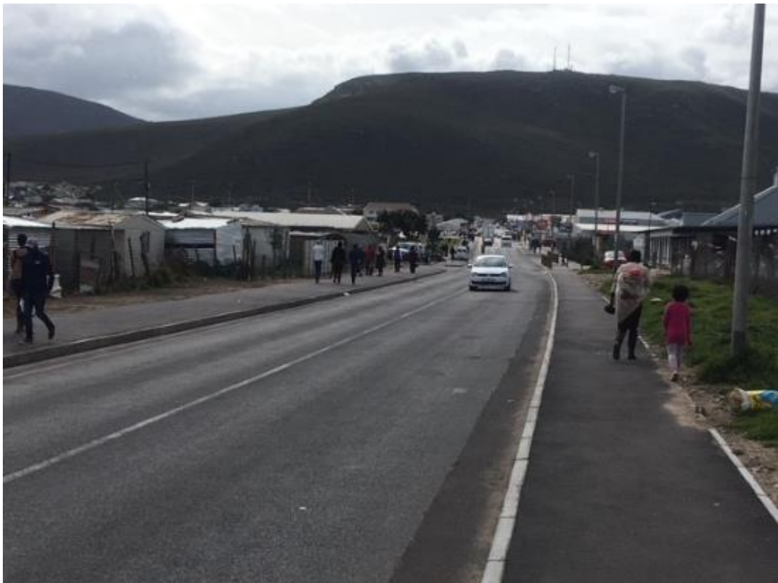
Figure 3-9 Before and After Swartdam Road NMT sidewalk installation
