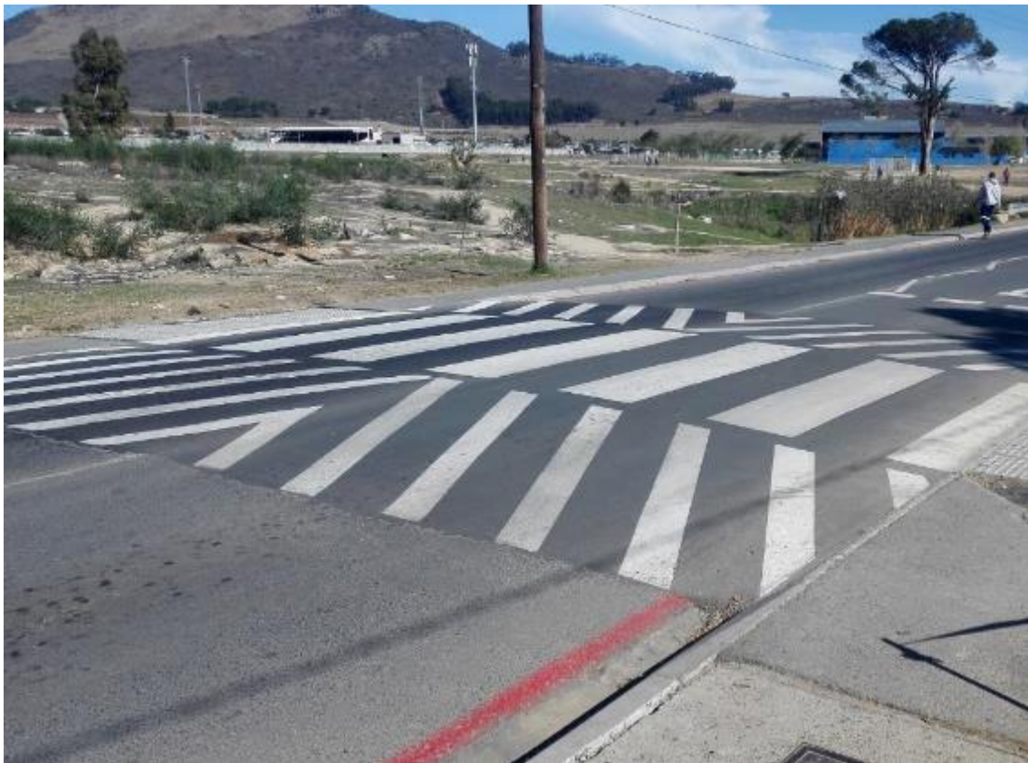
Figure 3-2 Pedestrian Crossing over Merchant Street Klapmuts
