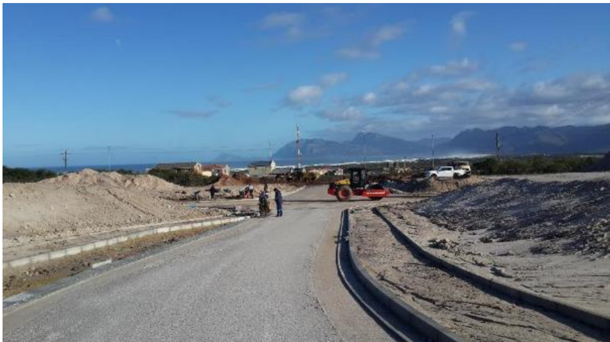
Figure 3-12 Hawston housing development – sidewalks under construction
