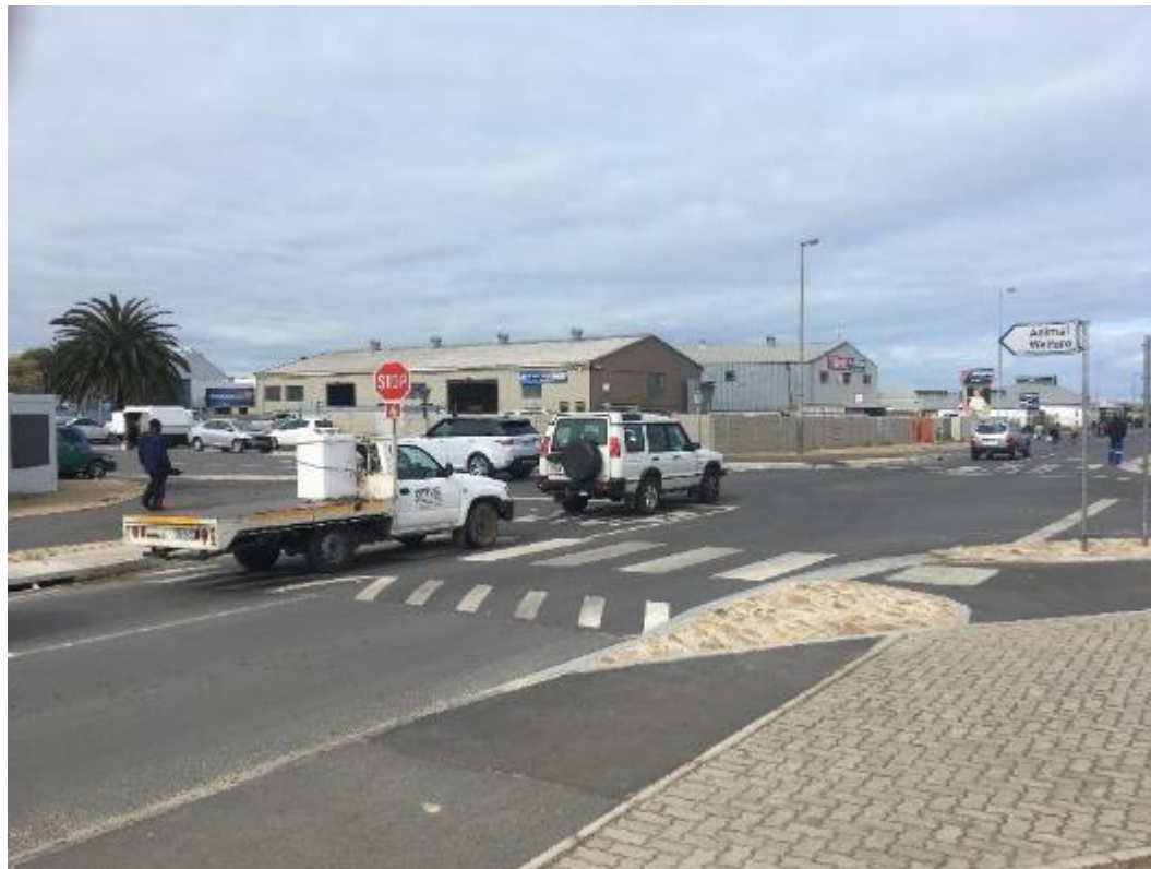
Figure 3-8 Before and After Steenbras and Swartdam Roads Intersection Upgrade
