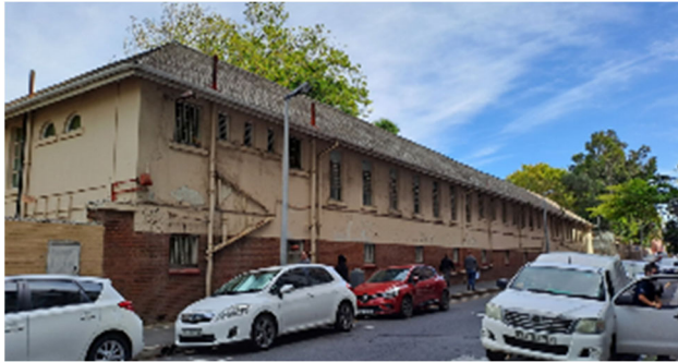
Prestwich Street facade
