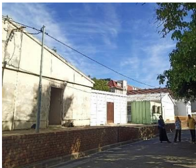
Outbuilding O/H line
