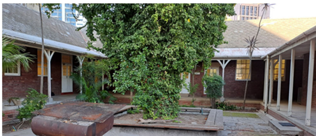
The verandah and courtyard of the Soils Lab
