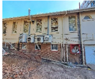
South-east façade of the Soils Lab
