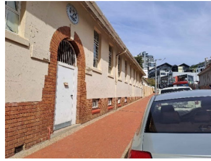
Original Main entrance on Chiappini Street
