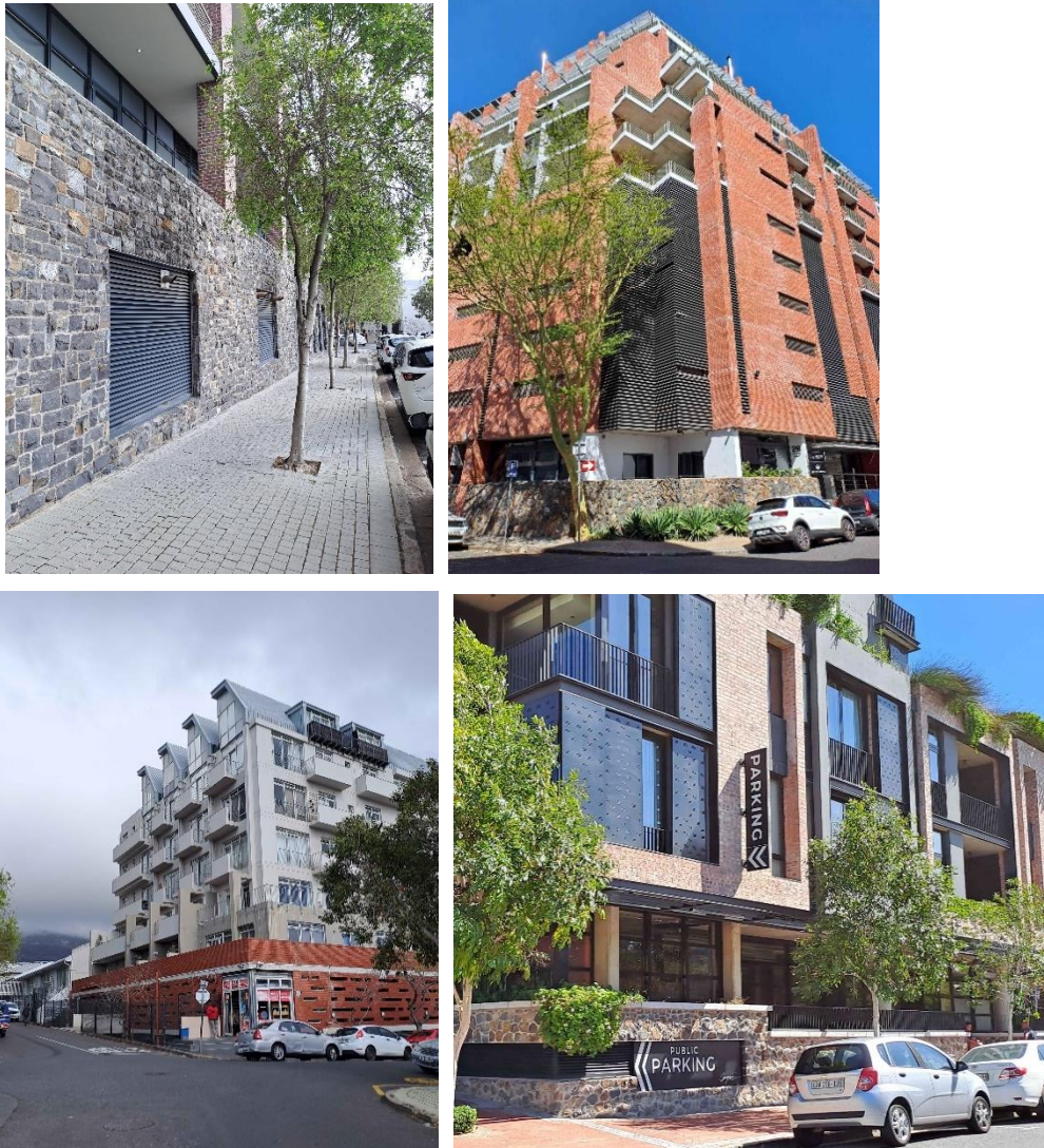
Figure 5.5: Examples of differentiating material of the ground floor and setting back the ground floor plane to break the vertical scale of the building (NM & Associates, 2023)
