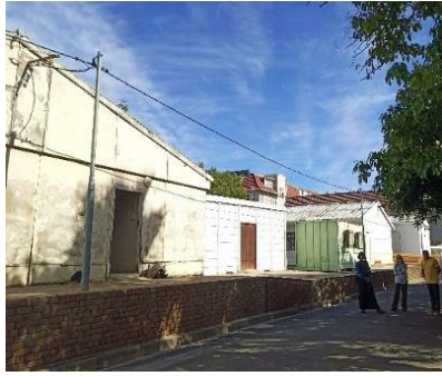
Outbuilding O/H line
