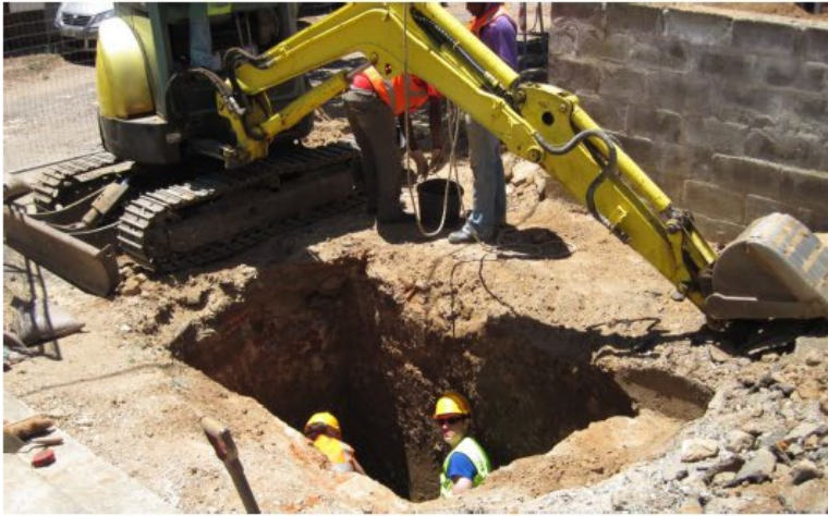
Figure 15 PTL 4 burial vault. The tomb was filled with very large shale boulders.
