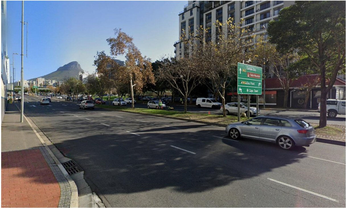
Figure 80: Existing view - Buitengracht Street looking west (Source: GE Streetview)
