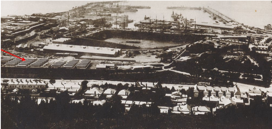
Figure 12: View of the Cape Town docks with the Docks Location, (arrowed) left (KAB AG951). To leave the Docks, workers would have to pass through the controlled Dock gates. Despite increasing restrictions on the movement of Africans there were still workers living in Districts One and Six. In District One many lived in the Jerry Street area. Despite crowded living conditions, living in the town was preferable to the controlled and regulated existence of the Docks Location. District One is situated to the right of the image.
