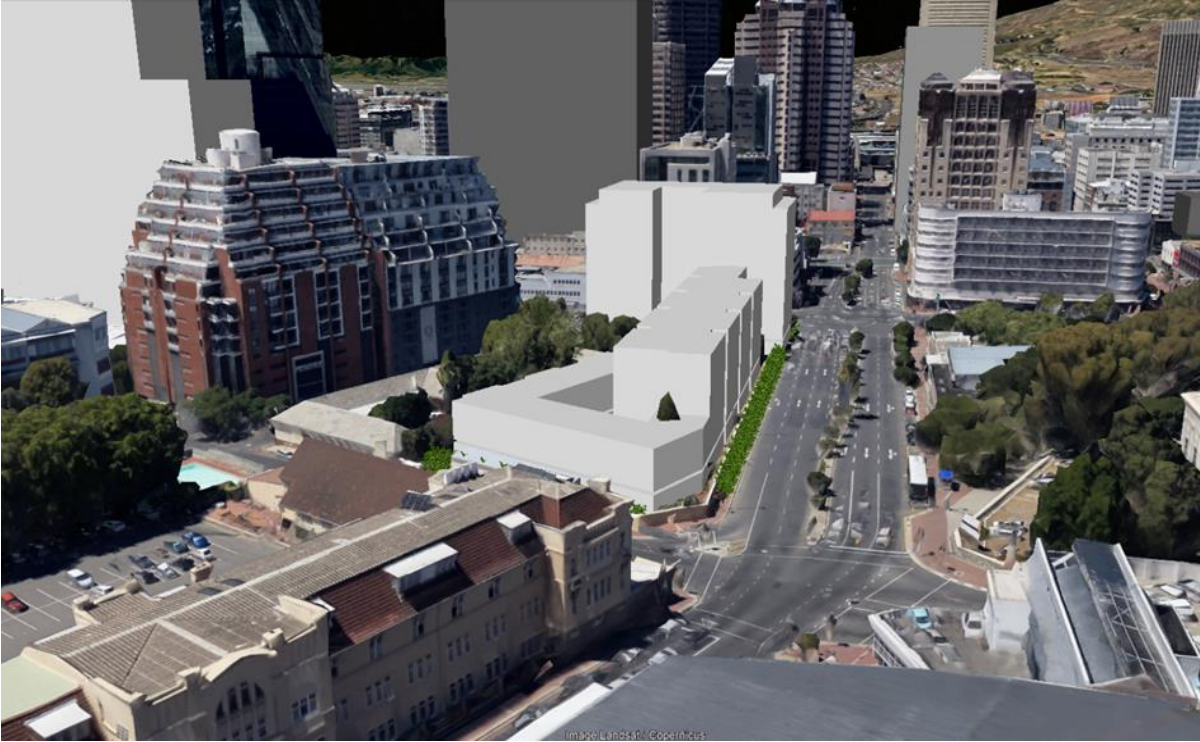
Figure 70: PPTL site (white), stepping down to the Salesian Institute (Sources: NM & Associates, GEPro)
