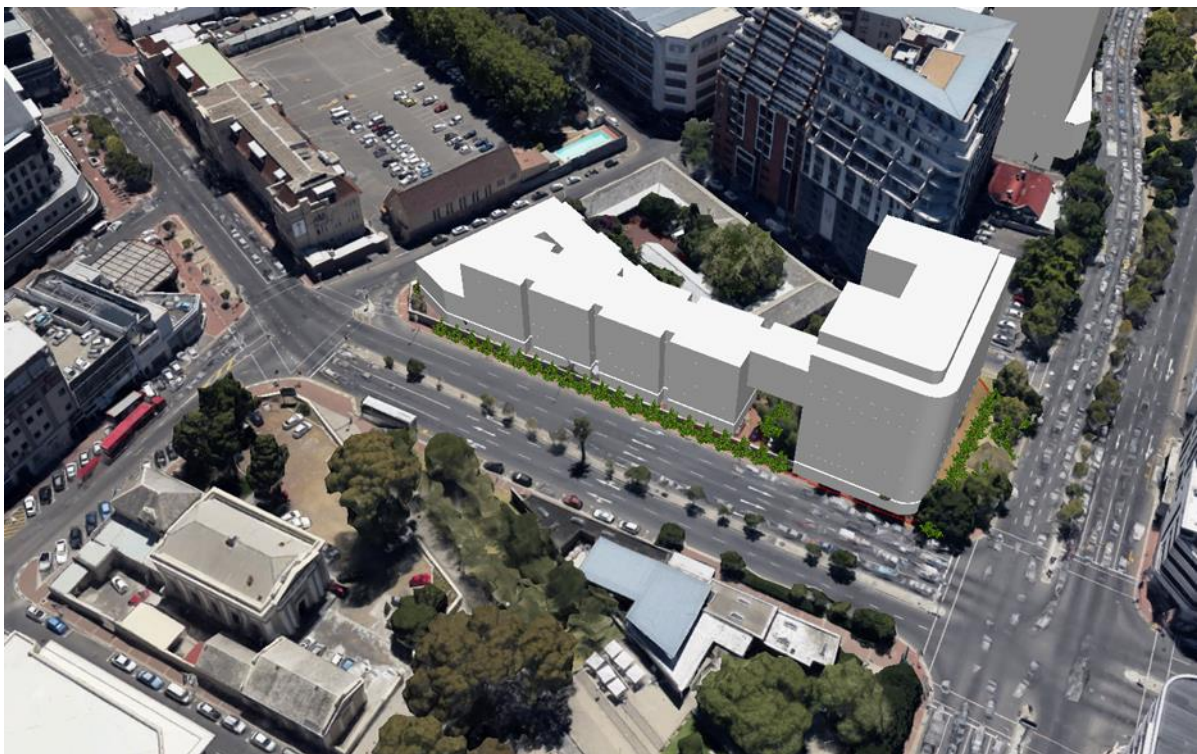
Figure 73: PPTL site (white) with tower at Buitengracht intersection (Sources: NM & Associates, GEPro)
