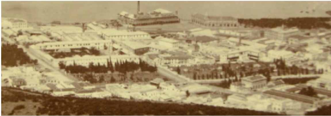
Figure 7. Date not known: DRC cemetery with walling, cypress trees and vaults on the inner north boundary (Source not known).
