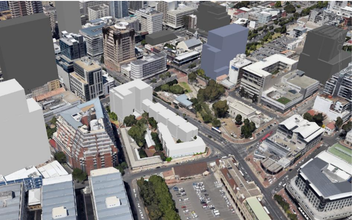
Figure 71: PPTL site (white) stepping down to the Soils Lab building (Sources: NM & Associates, GEPro)
