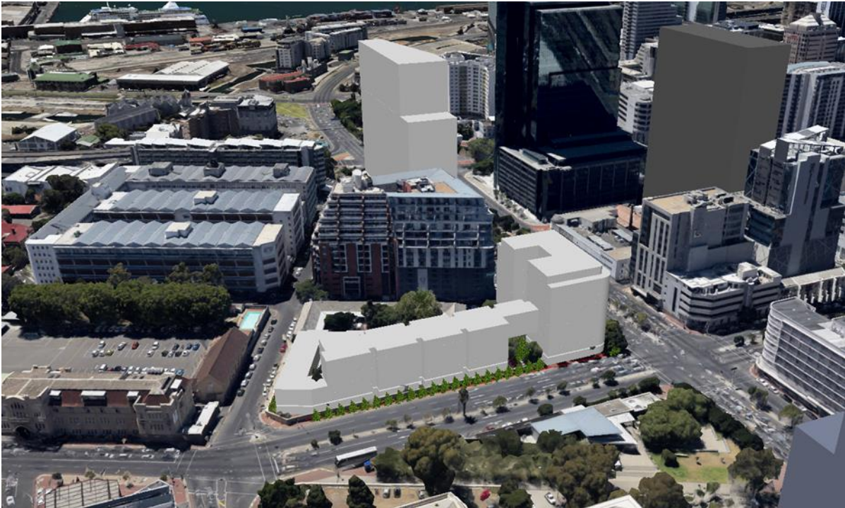
Figure 72: PPTL site (white), with trees along Somerset Road (Sources: NM & Associates, GEPro)
