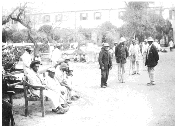
Figure 64. The Old Somerset Hospital. This was the central courtyard around which the dormitories were arranged. The Annex building eventually became U-shaped, around which rooms were arranged with a central space for oversight. (Worden et al., The making of a City 1998.)
