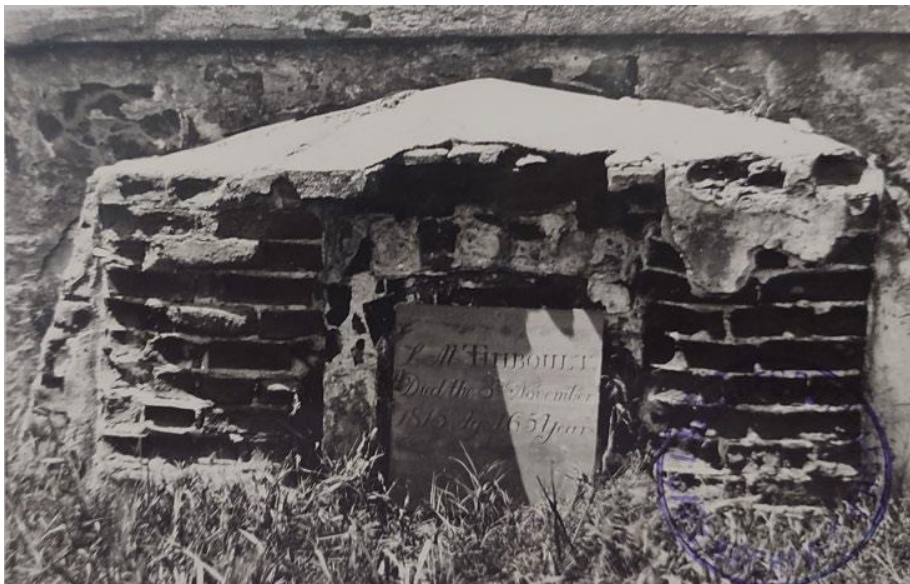
Figure 61: The vault of the Thibault family. The tombstone is for L M Thibault who is recorded as dying on 3 November 1815 aged 65 years. While the condition of the vault has deteriorated in this photograph, it was known to have been to the design of Schutte, also buried in the cemetery. A note attached to the photograph reveals that it was situated inside the walls but close to the Buitengracht Street pavement. This means it was disturbed during the Buitengracht Street road widening. (E 3939.) Vaults were above ground and when the site was exhumed the vaults were demolished and the human remains removed.
