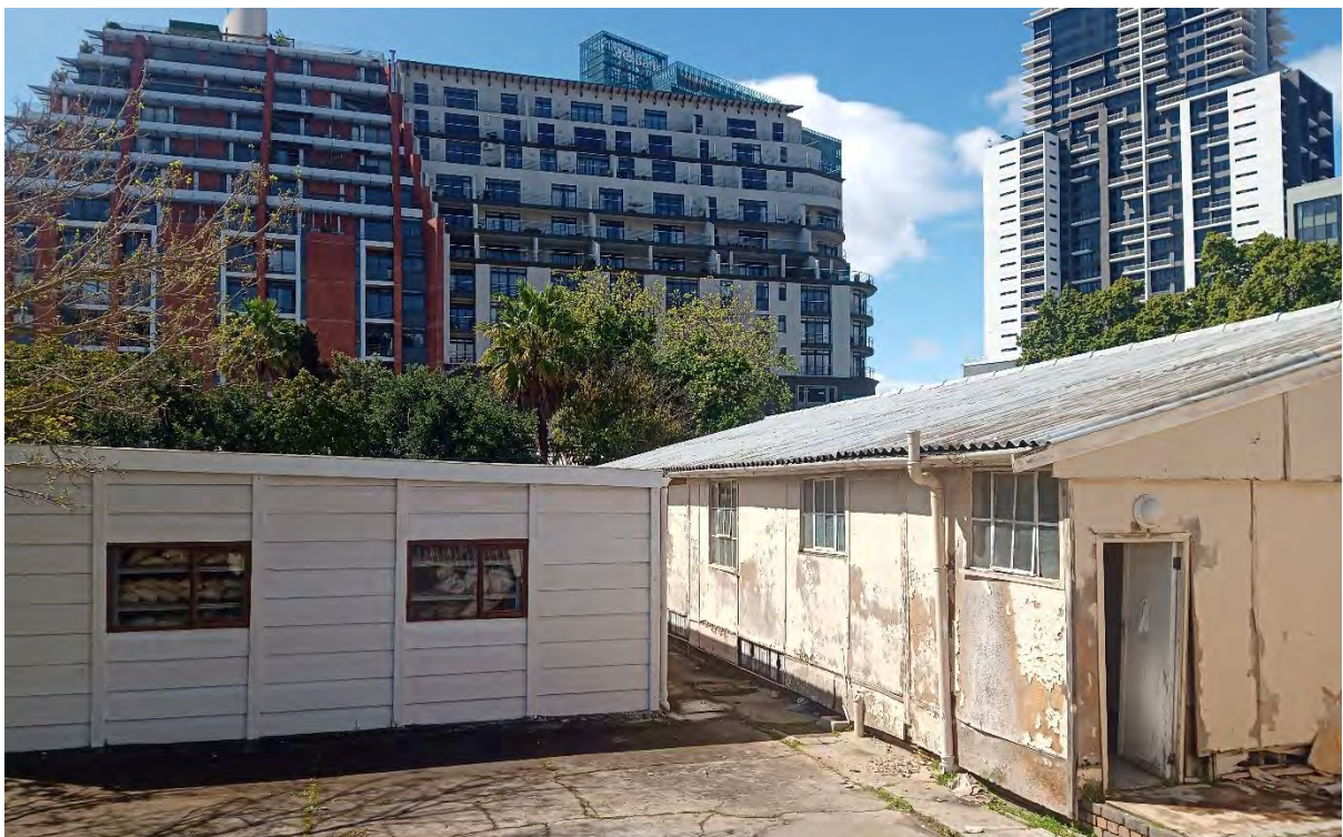
Figure 72: Existing prefabricated structures on site (proposed to be demolished).
