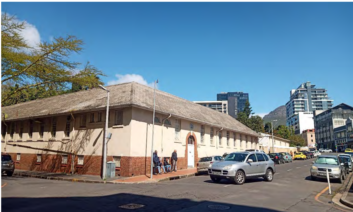
Figure 64: Prestwich Street / Chiappini Street corner, showing Soils Lab doorway.
