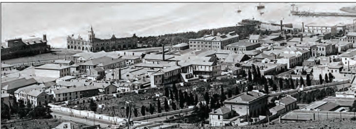
Figure 6. The DRC cemetery c1900 showing positioning of vaults against the boundary walls and down the centre of the long axis. This photo pre-dates the exhumation (Wilson 2023:3 Michael Fortune collection).
