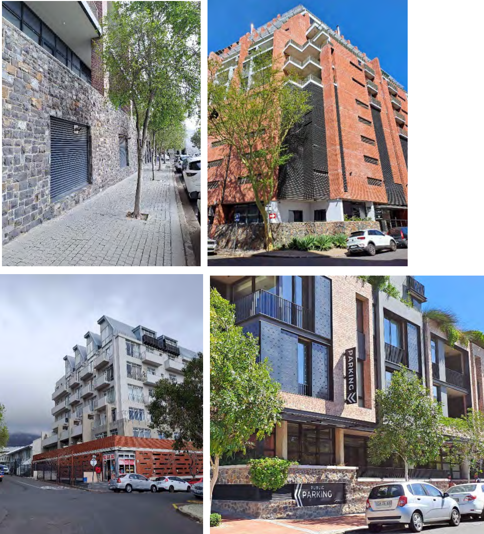
Figure 3.6: Examples of differentiating material of the ground floor and setting back the ground floor plane to break the vertical scale of the building (NM & Associates, 2023)
