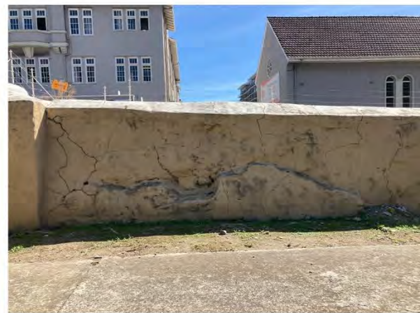
Remaining historic walling on Chiappini Street
