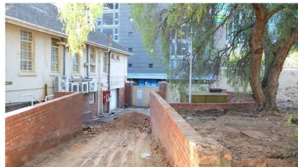
Closed entrance from site to Prestwich Street
