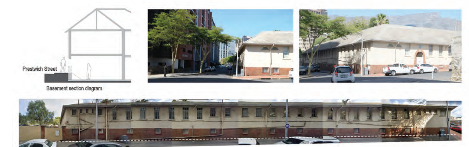
Soils Lab Prestwich Street Elevation (Source: Winter, 2024)
