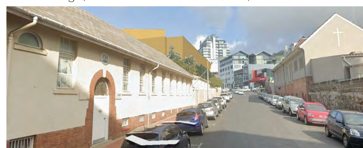
Soils Lab (Chiappini Street façade) simulation: proposed development (yellow) just visible. (Sources: NM&A, GEPro in Gibbs, 2024)
