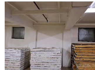
Soils Lab Basement, with window openings to Prestwich Street
