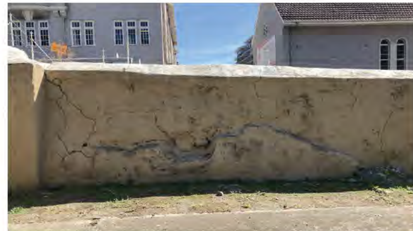
Figure 29. Chiappini Street old walling viewed from within the site (photo 04-2023)
