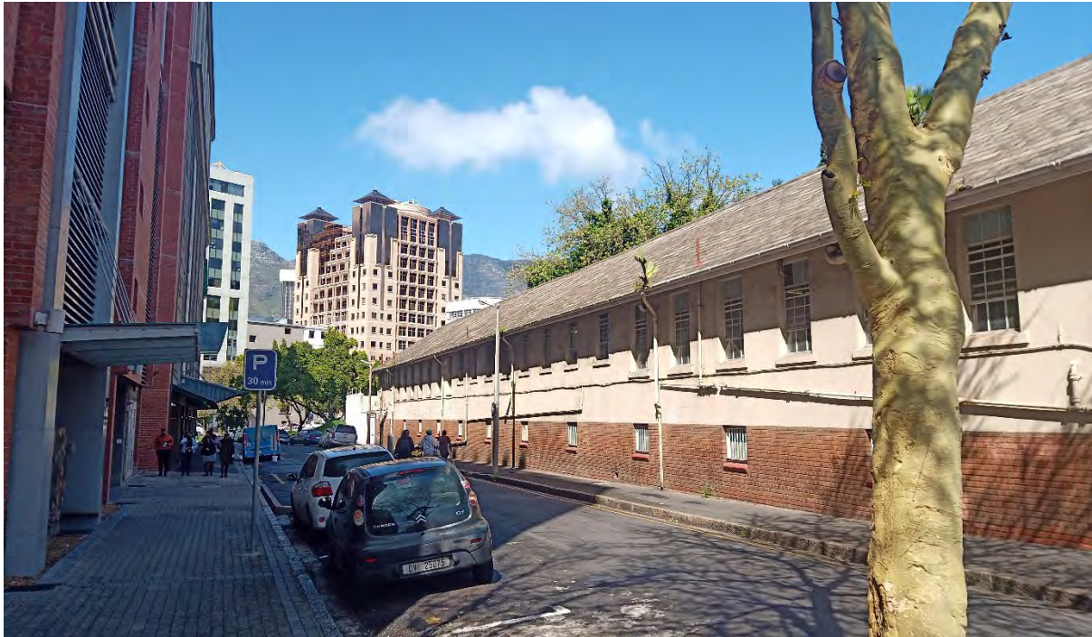
Figure 63: Soils Lab building – Prestwich Street elevation. (note lack of active interfaces).
