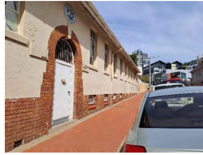
Original Main entrance on Chiappini Street
