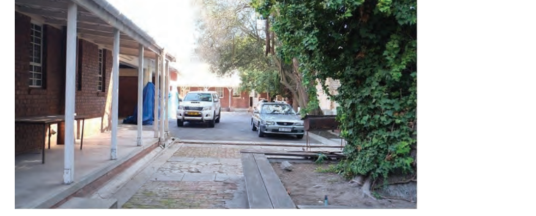
24. Soils Lab Building courtyard interior views (NM&A, 2024)
