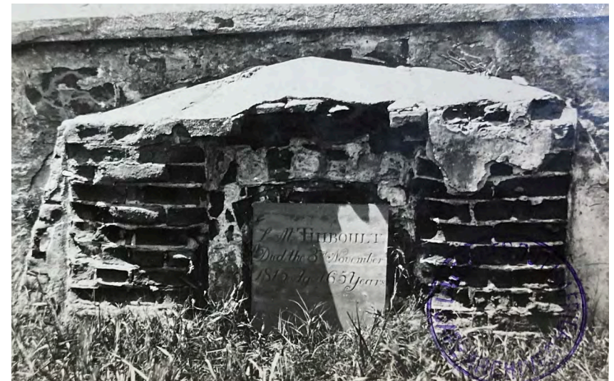
Figure 11. Example of built fabric: Tomb of LM Thibault, according to archive note this is now located below Buitengracht Street pavement. (KAB E3939).
