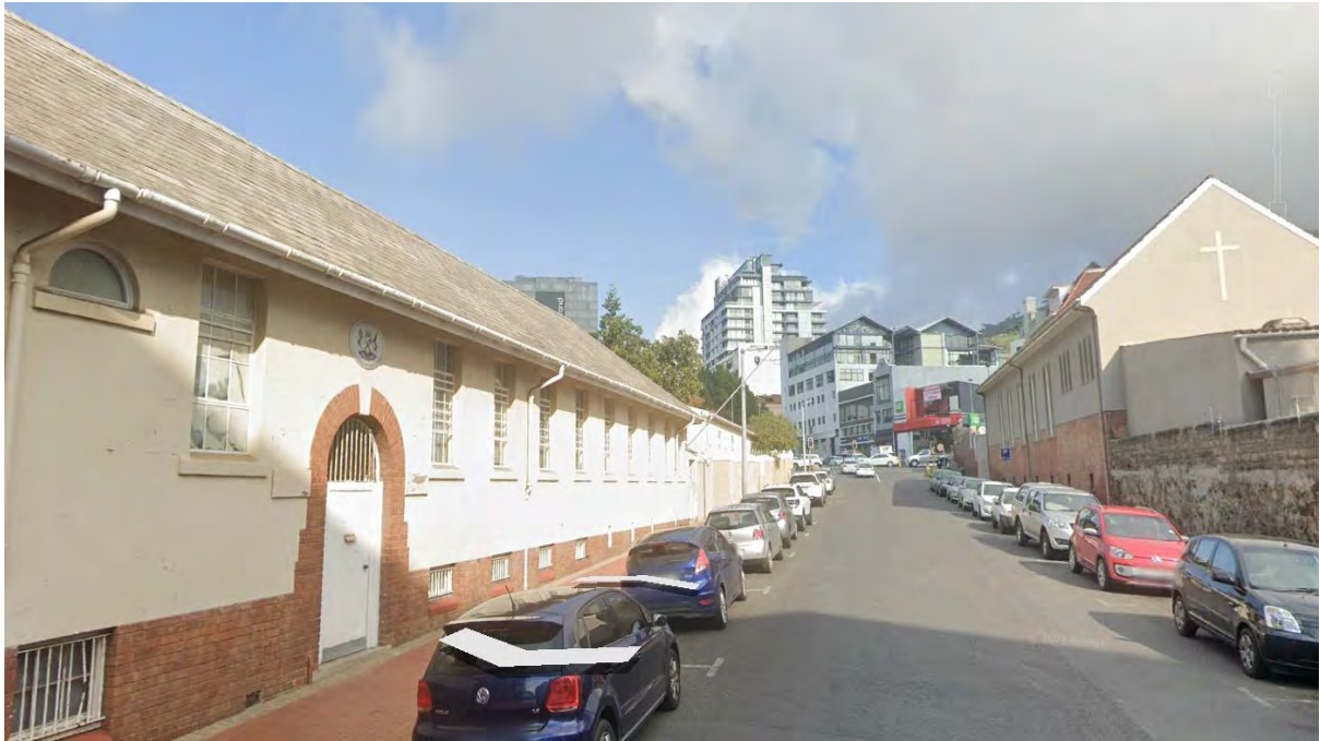
Figure 86: Soils Lab (Chiappini Street façade): existing view (Source: GE Streetview)
