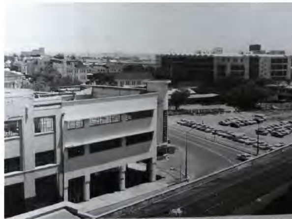
Figure 16. Reference: 1974 Robb Motors building - demolition for road widening. (KAB CA839)
