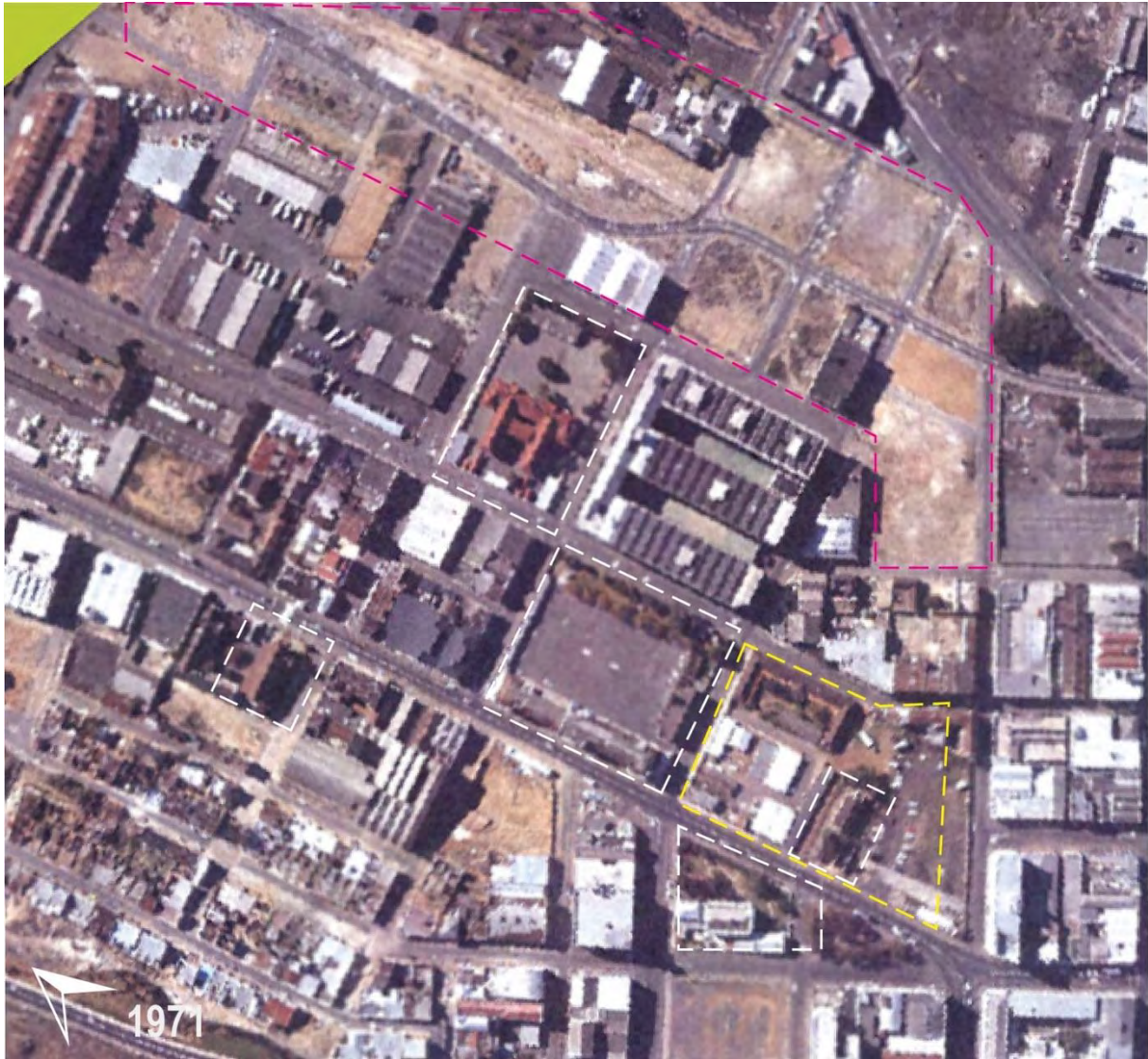
Figure 39: 1971: Prestwich School, St Andrew's, St Stephen's and Sacred Heart Churches and the Salesian Institute remain (white outline); demolition and clearing to make way for Western Boulevard (pink outline). (Source: CoCT Map Viewer)
