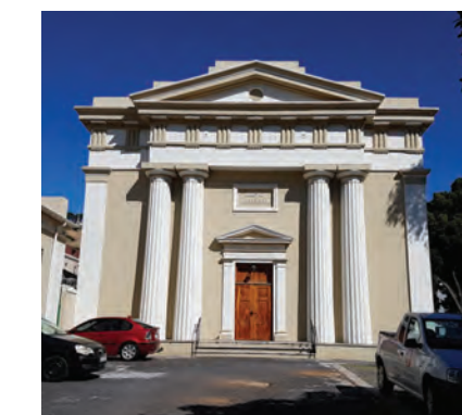
St Andrew's Presbyterian Church on Somerset Road.
