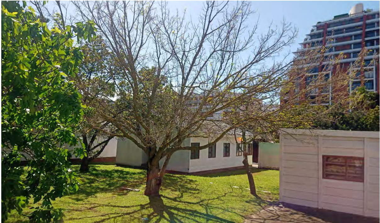
Figure 71: View into the site from the Somerset Road site access gate.
