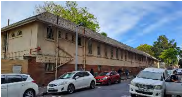
Prestwich Street facade
