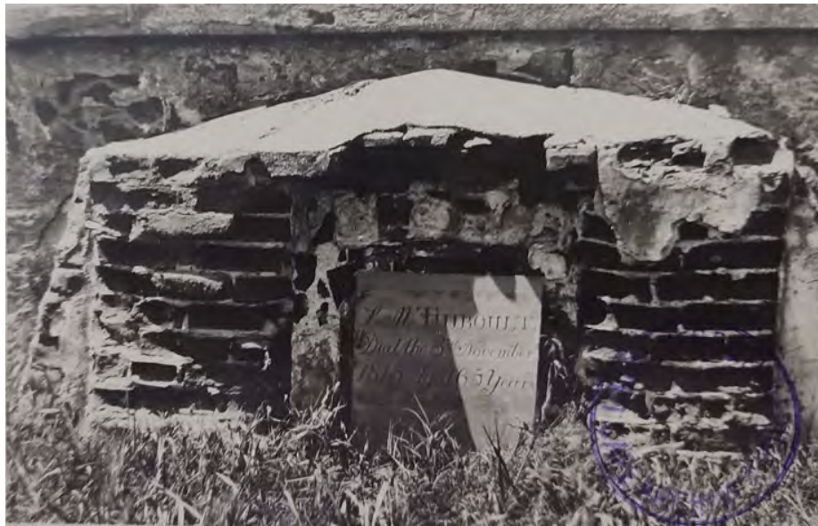
Figure 41: The vault of the Thibault family. The tombstone is for L M Thibault who is recorded as dying on 3 November 1815 aged 65 years. While the condition of the vault has deteriorated in this photograph, it was known to have been to the design of Schutte, also buried in the cemetery. A note attached to the photograph reveals that it was situated inside the walls but close to the Buitengracht Street pavement. This means it was disturbed during the Buitengracht Street road widening. (E 3939.) Vaults were above ground and when the site was exhumed the vaults were demolished and the human remains removed.
