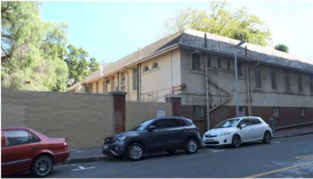
15. Site entrance (bricked closed) off Prestwich Street
