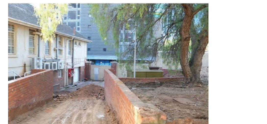
25. Closed entrance on Prestwich Street (Winter, 2024)
