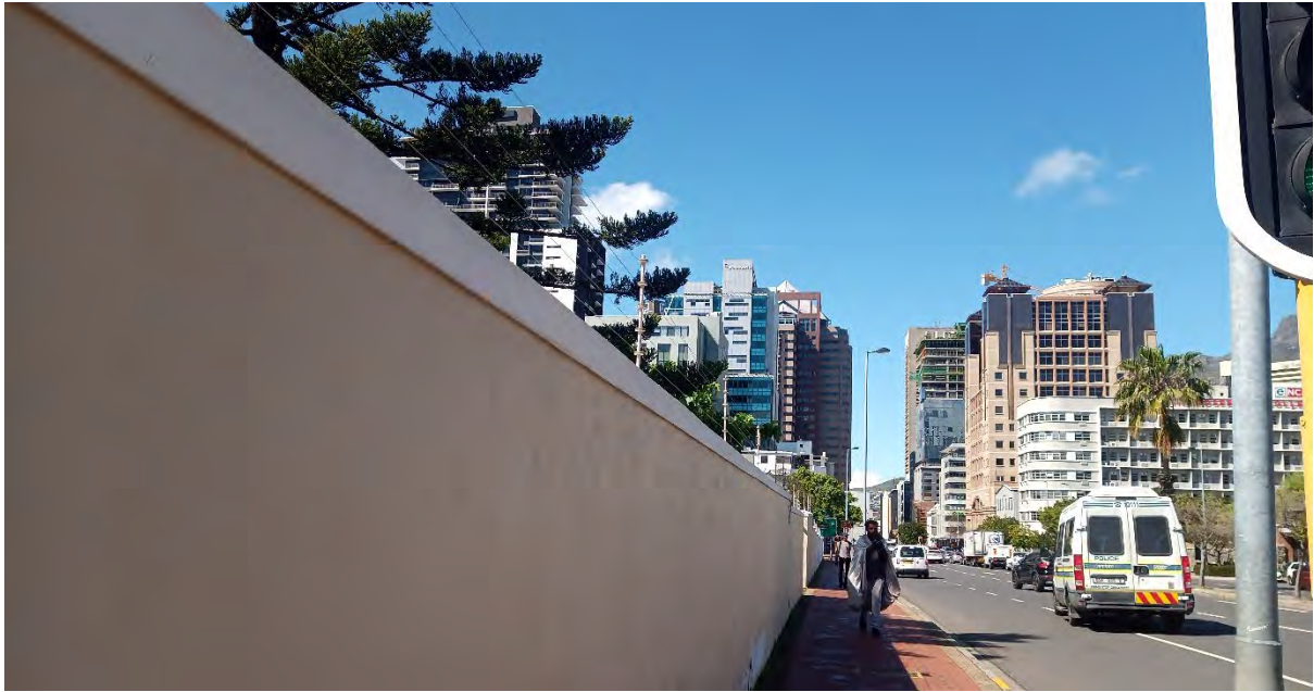
Figure 69: Somerset Road interface: existing wall and inactive site edge.
