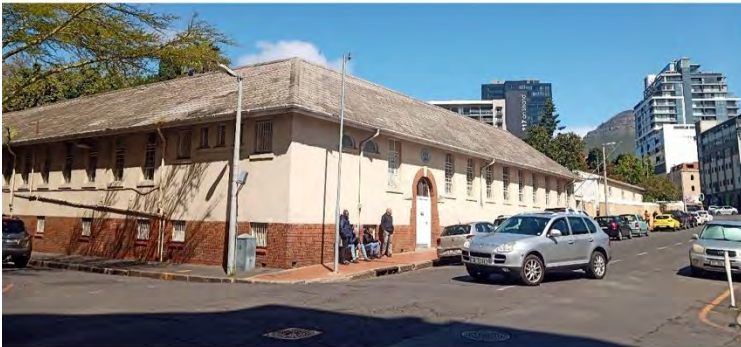
17. Prestwich-Chiappini Streets intersection, entrance to Soils Lab building (Gibbs 2024)
