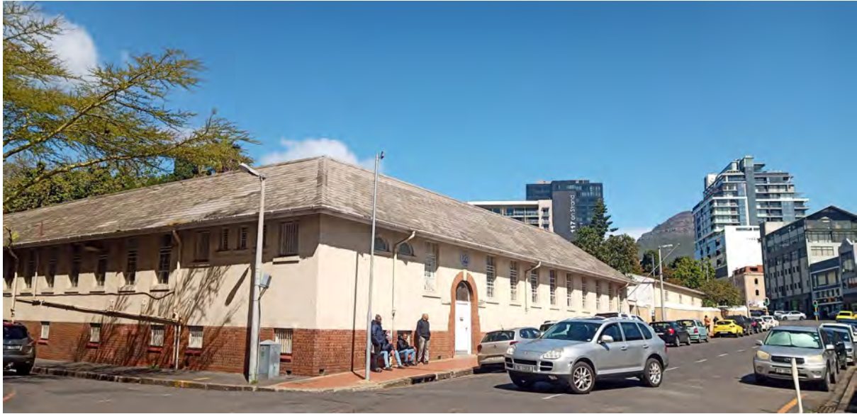
Figure 6: The Soils Lab building with Lions Head in the background
