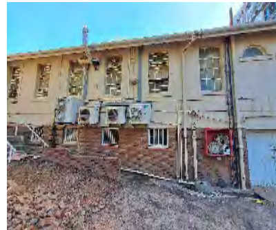
South-east façade of the Soils Lab
