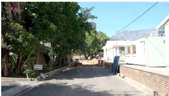
Entrance to site off Chiappini Street
