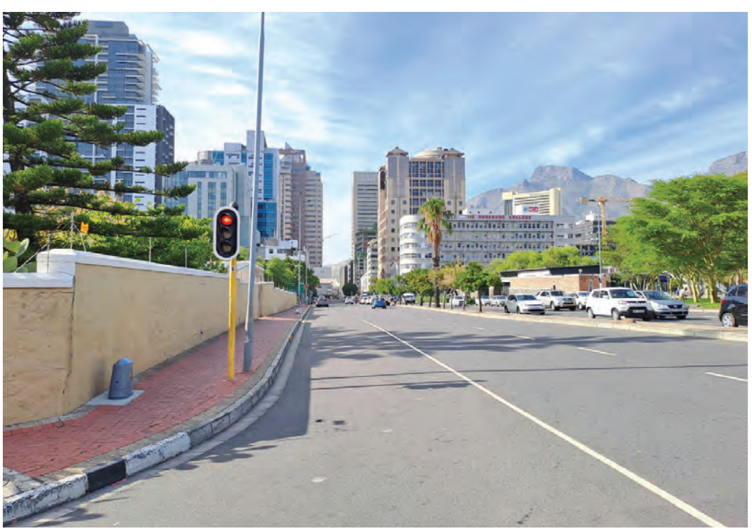
4. Somerset Road view south-east (NM&A, 2023)
