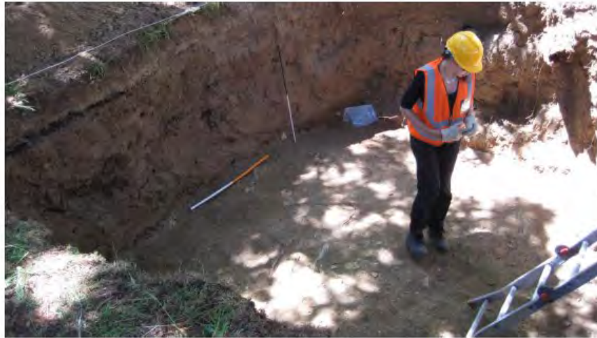
Figure 4. Excavation PTL 1 was a generous sized hole located towards the south west side of the erf among trees behind the prefab structures. This image depicts the excavation at the point at which bedrock is reached. The deposits were highly disturbed, and contained very little articulated bone.
