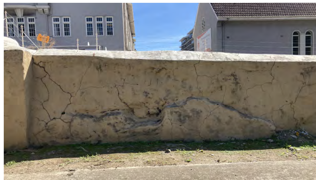
Figure 29. Chiappini Street old walling viewed from within the site (photo 04-2023)
