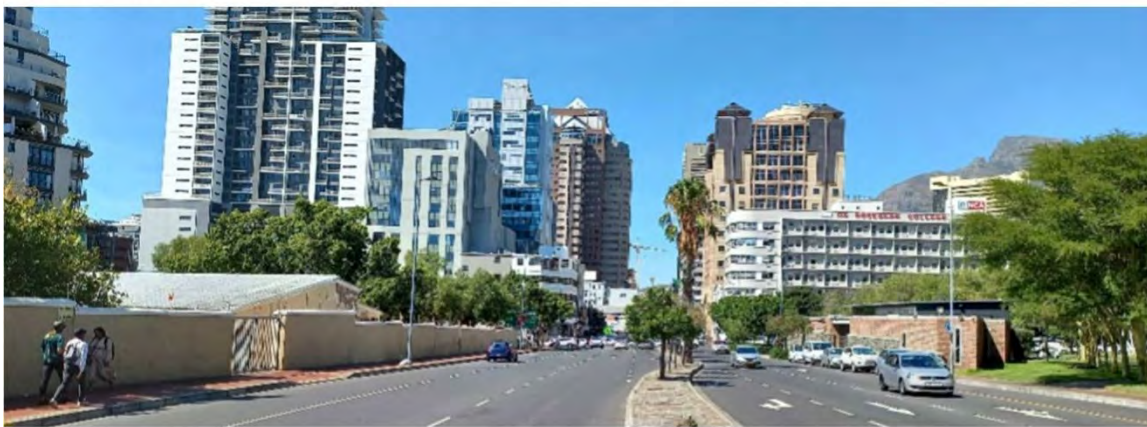
1. Somerset Road view east (NM & Associates Planners and Designers)
