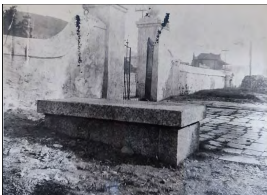
Figure 40: The tombstone of Andrew Barnard, who died in 1807. In the distance beyond the Somerset Road entrance gate is the Masonic Lodge Tomb, which was among the plots numbered 72 to 75, owned by the Lodge (Schultz; KAB AG 10).
