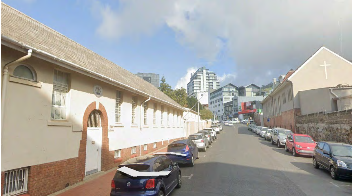
Figure 103: Soils Lab (Chiappini Street façade): existing view. Source: Streetview
