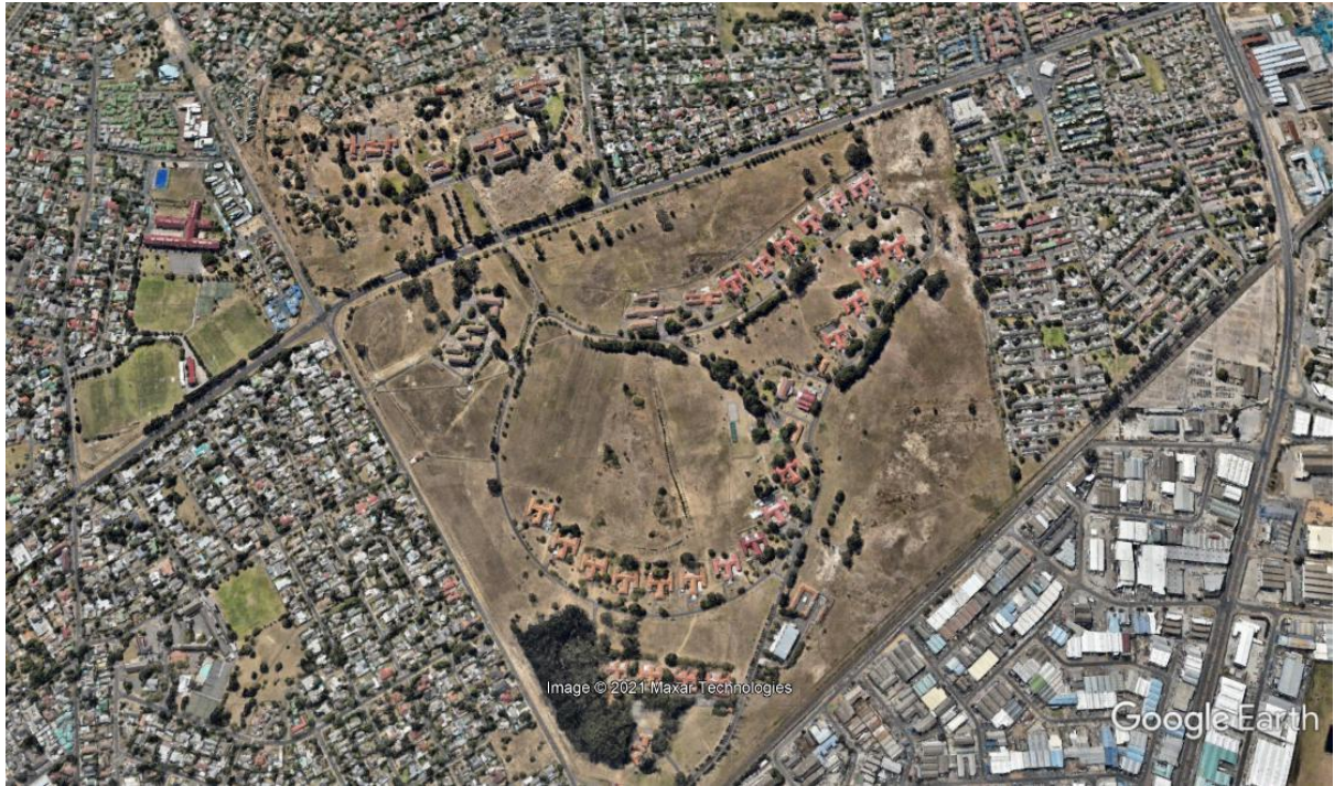
Figure 7.7-23 Stikland Psychiatric Hospital site (Google image 2021), virtually unchanged since it was constructed
