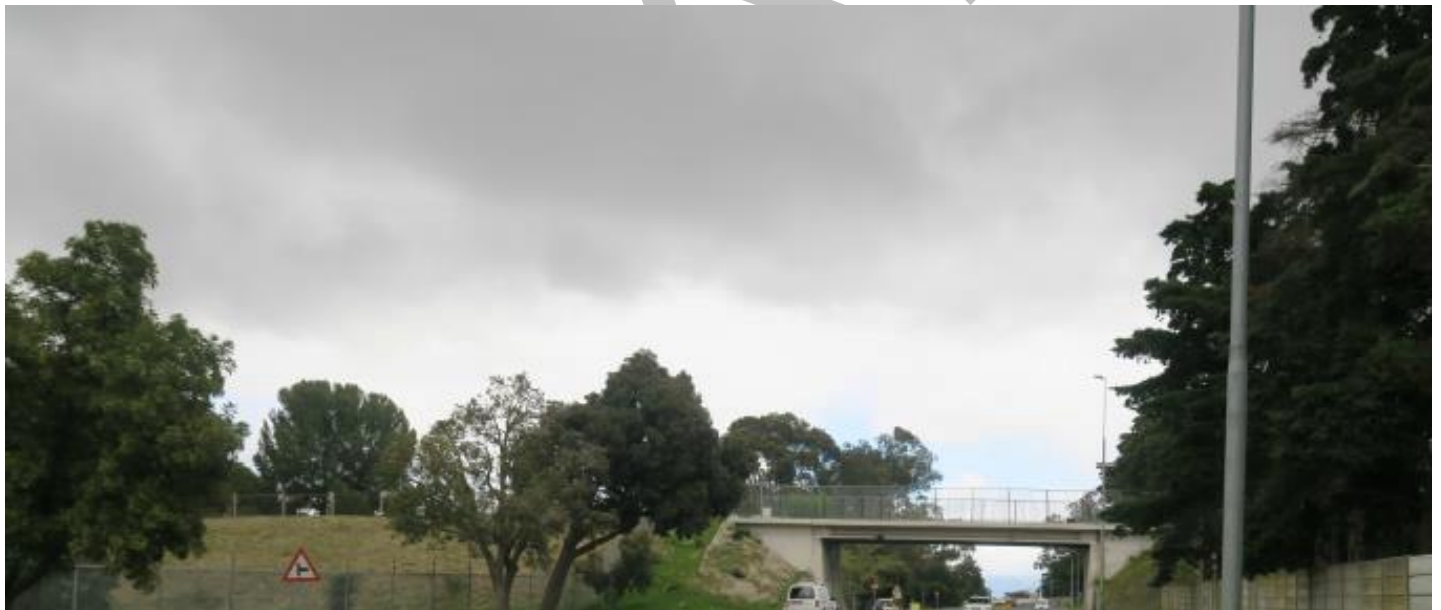
Figure 7.7-31 The R301 as it passes through Stikland Hospital, Stikland South to the left; Stikland North to the right, the disused bridge connecting the two
