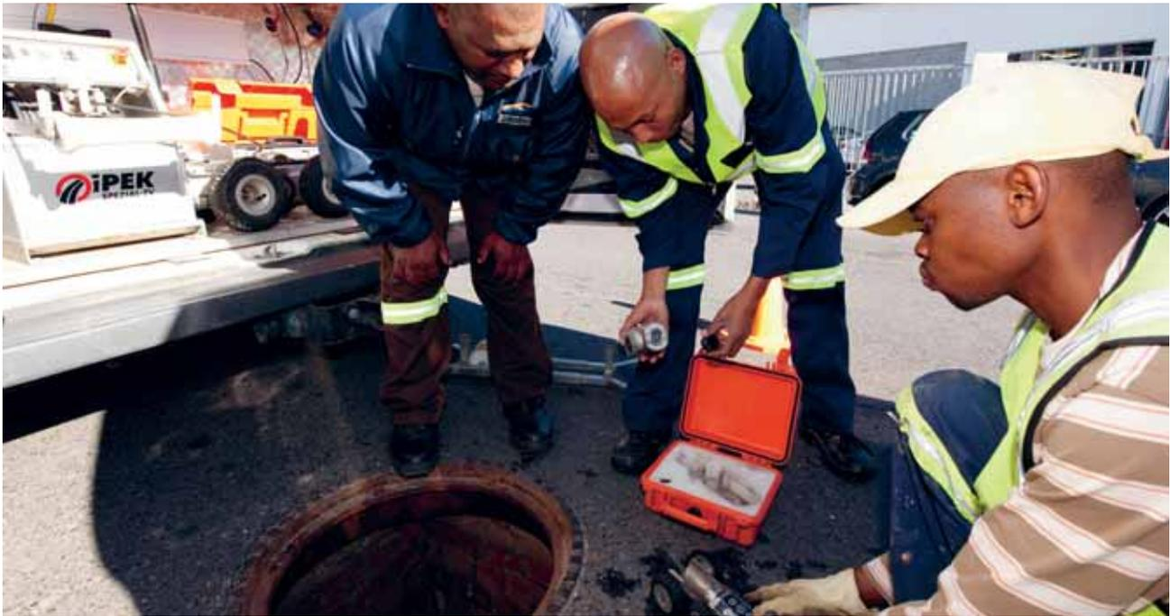
City staff using closed-circuit television (CCTV) inspections to enhance proactive sewer maintenance
