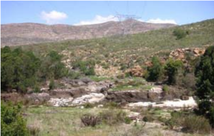
Figure: Erosion & wetland disturbance at the Kliprivier along Outeniqua pass
