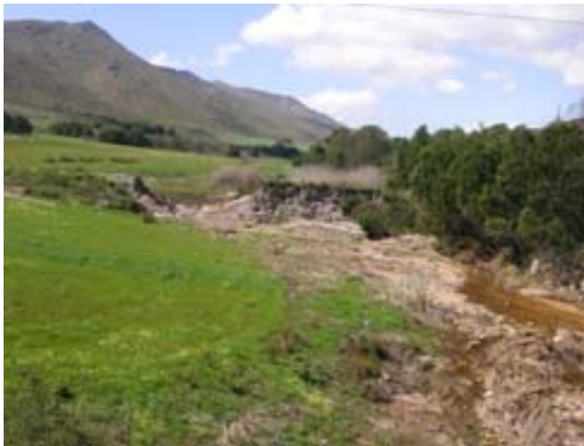
Figure: 4.2.7e Dam wall break at the Kliprivier, with associated wetland disturbance
