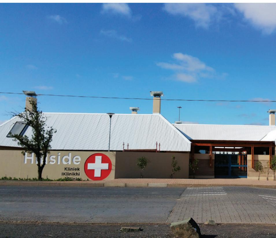
The new Hillside Clinic in Beaufort West contains the most “green” features of any primary healthcare facility in the Western Cape. Rammed earth walls and underground rock stores reduce the need for air conditioning by mitigating temperature extremes (high temperatures during the day, and cold temperatures at night). The design also features optimised natural daylight, energy-efficient light fittings, solar water heating, and a borehole for irrigating the water-wise garden.
