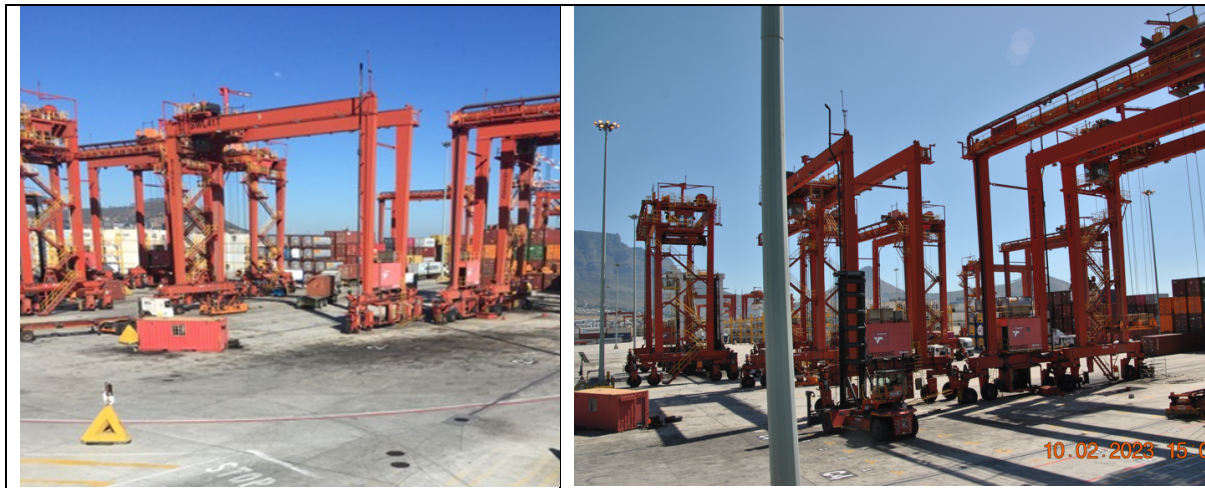
Figure 82: Cranes awaiting repairs
