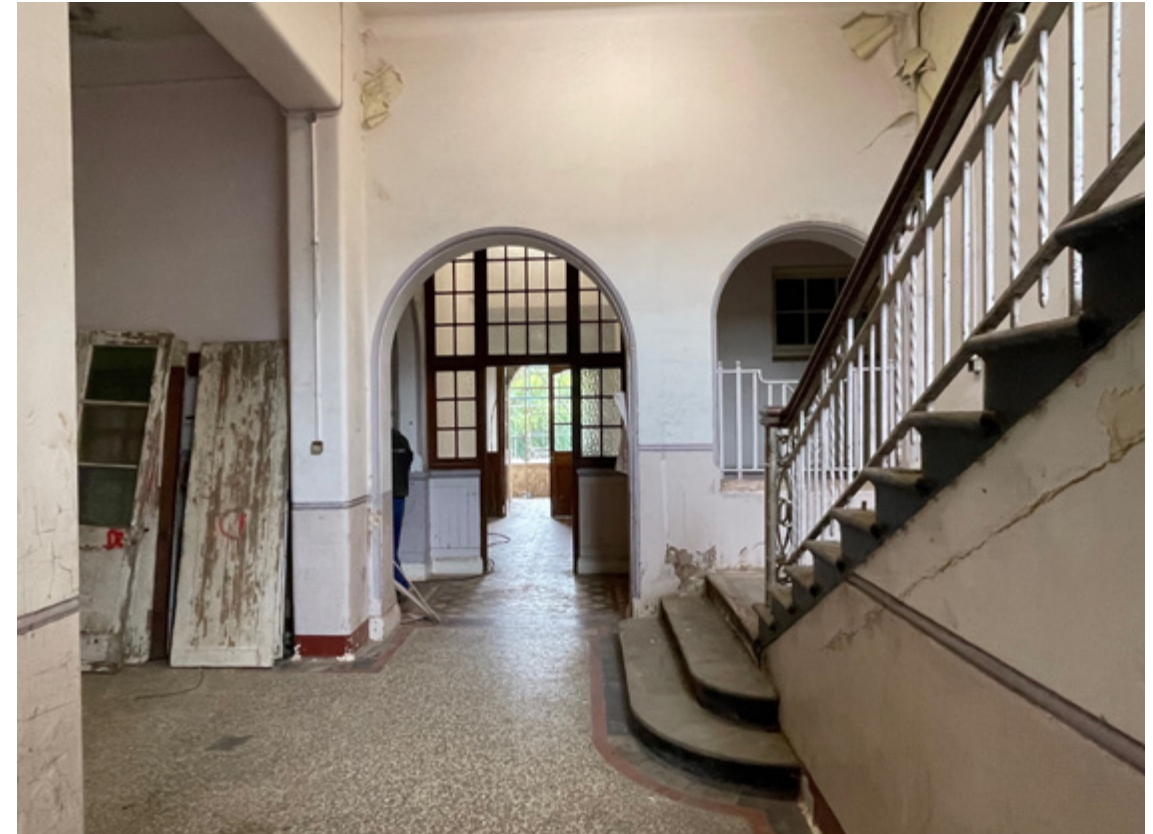
Figure 94. RSA (2023) 1913 school building staircase lobby with a view of the original building entrance.
