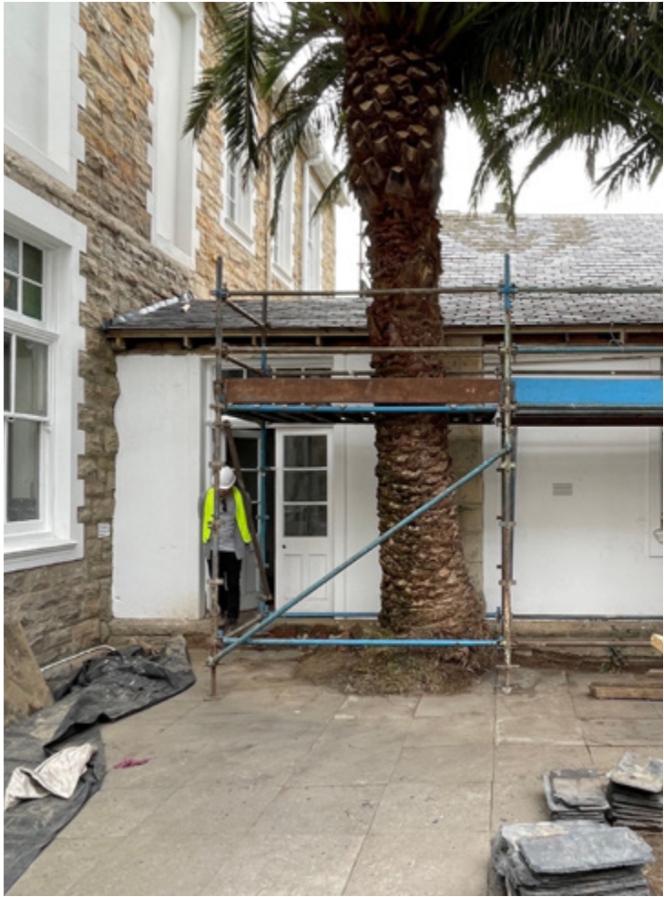
Figure 112. RSA (2023) Junction between the 1901 building and the 1905 Extension.
