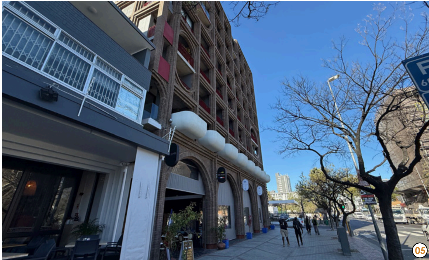
Figure 182. RSA (2025) Main Rd pavement adjacent to a newly developed 21st-century residential building replacing 2-3 story mixed-use commercial structures with some architectural merit. New development with a good street interface, contributing greatly to the evolving streetscape and context
