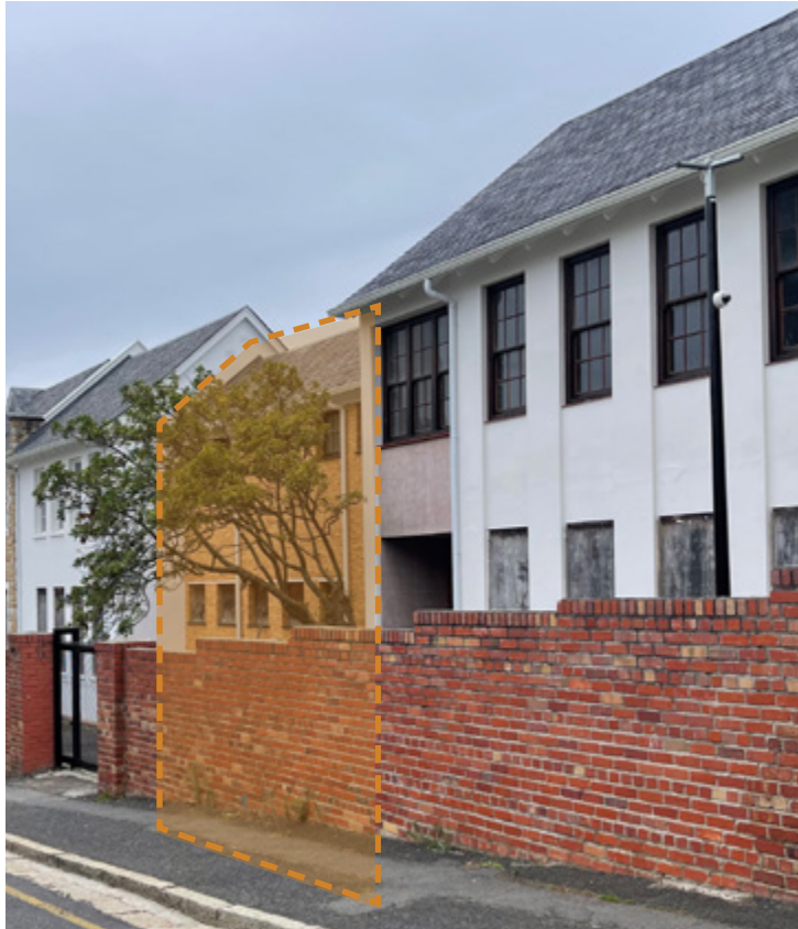
Figure 141. RSA (2023) c.1970 Ablution Facilities Additions, from The Glen.
