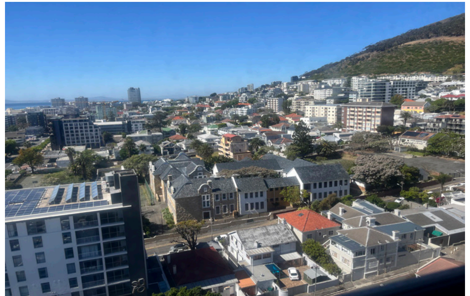
Figure 67. RSA (2023) Building scale difference between the lower part of Sea Point and the higher part, closer to the mountain.
