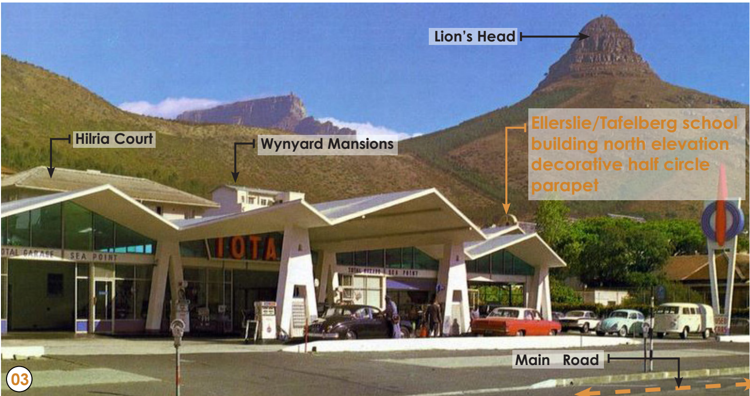
Figure 171. RSA (2025) The Total garage on the corner of Main and Milner Rds, with a magnificent triangle profiled concrete forecourt roof 1968, replaced with a conventional steel roof. (After - Etienne du Plessis - flickr.com)
