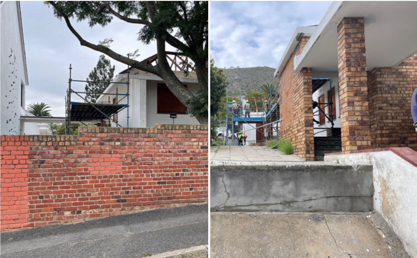
Figure 147. RSA (2023) Concrete-covered walkway leading to the music building's entry portico.
