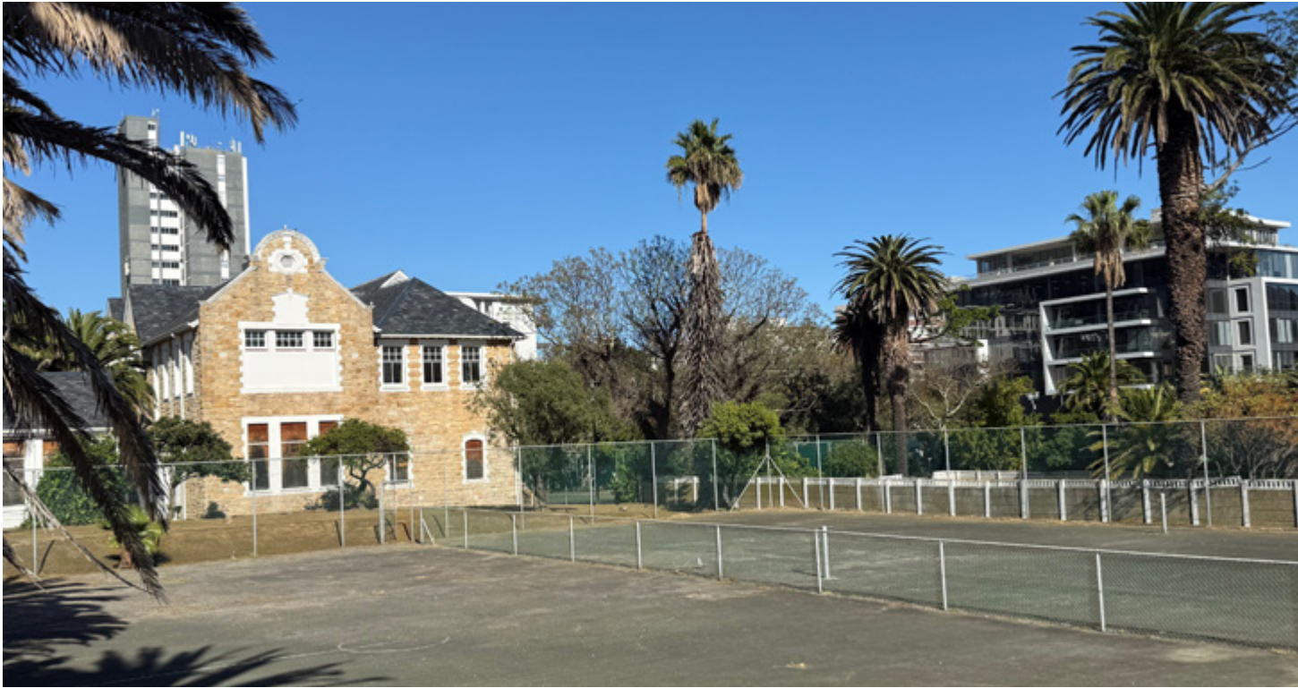
Figure 153. RSA (2025) View from Milner Rd looking at the Tennis court in front of the school building's northeast façade.
