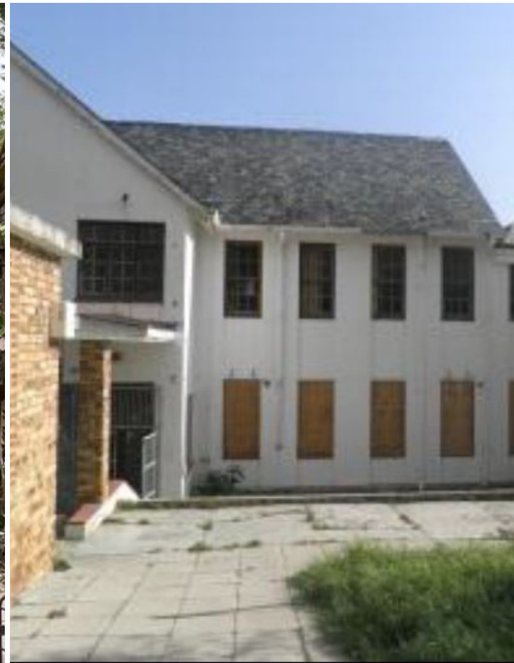
Figure 144. Bridget O'Donoghue (2011) c.1970 Double-storey Classroom Additions, viewed from the Music Building.
