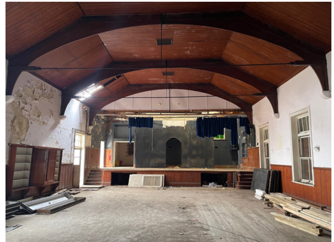
Figure 95. RSA (2023) School hall interior facing the stage.
