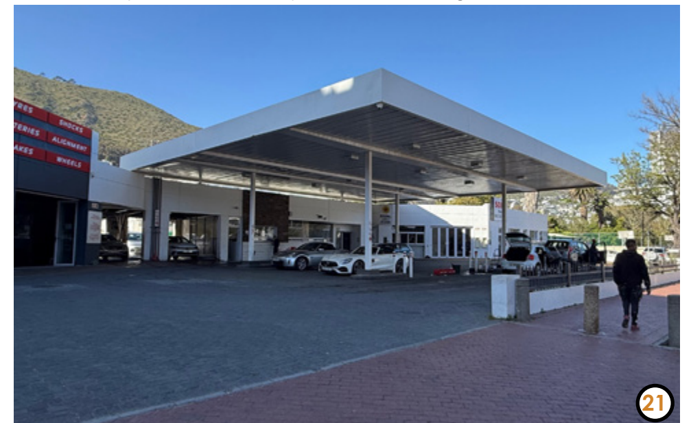
Figure 24. RSA (2025) Late 20th-century petrol station, old forecourt roof replaced.
