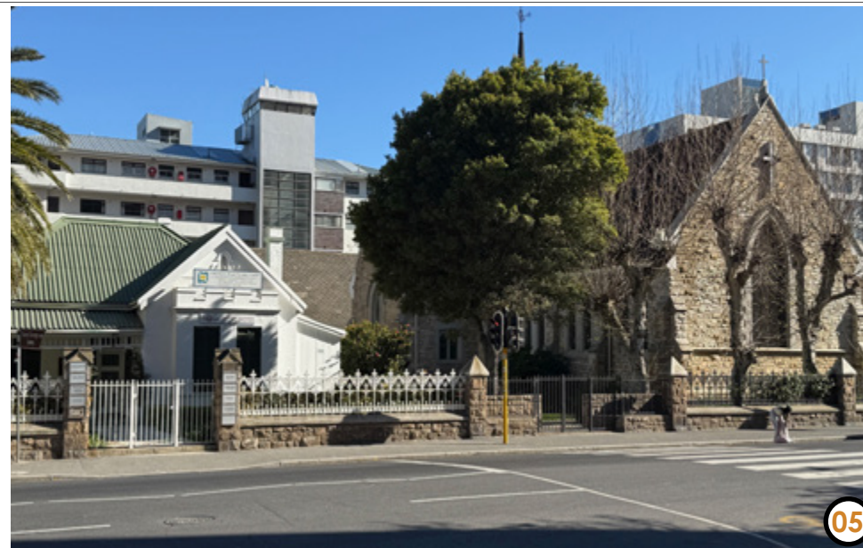
Figure 14. RSA (2025) Evangelical Congregational Church, to the left, residential property part of the site still intact. 05
