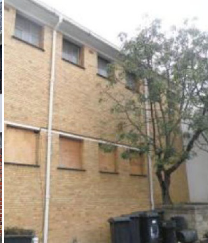
Figure 142. RSA (2023) c.1970 Ablution Facilities Additions, facebrick facade.
