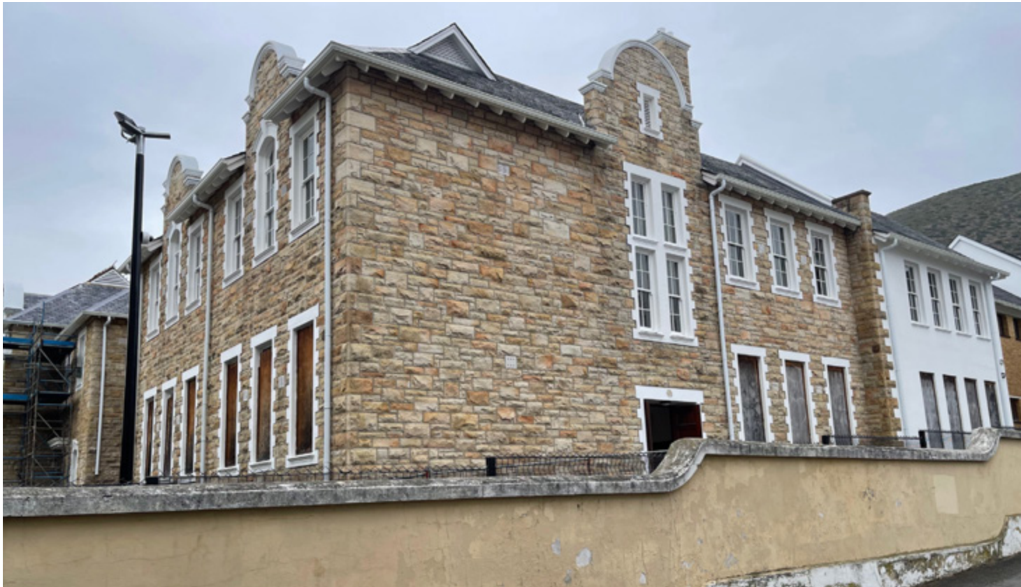
Figure 118. RSA (2023) 1936 Double Storey School Building from The Glen Road.
