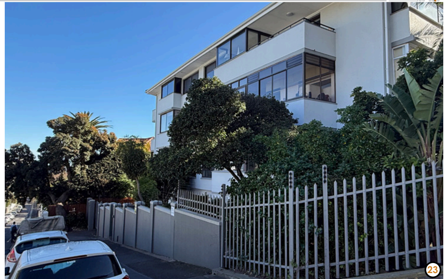
Figure 58. RSA (2025) Glenlyn Court from High Level Rd, Conner High Level Road, and The Glen.
