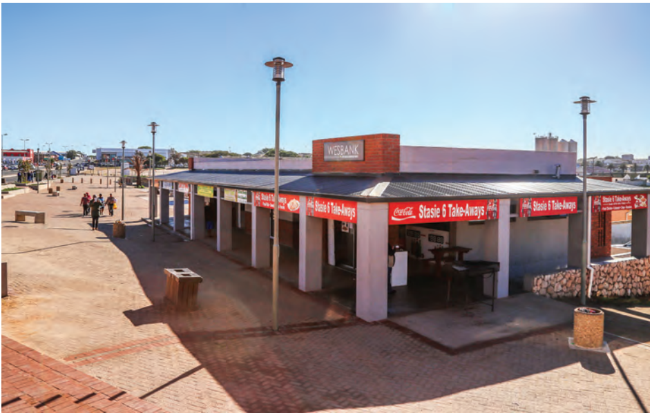
Figure 15: LED units in Wesbank
