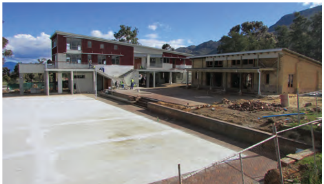
Figure 28: Resource Centre under construction
