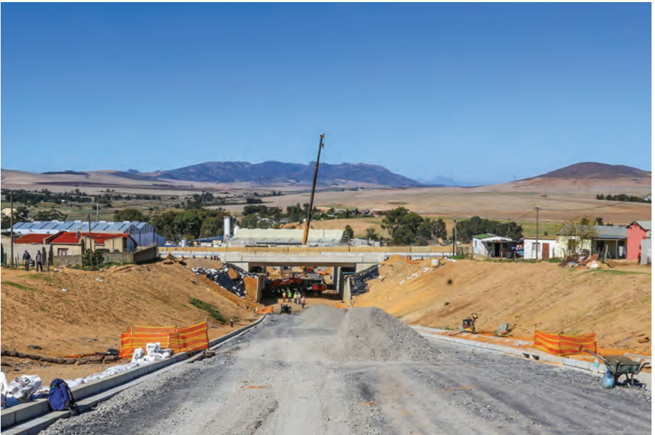
Figure 18: SANRAL underpass with additional paved and safe pedestrian pathway
