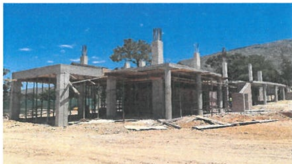
Figure 6: Villiersdorp Resource Centre Construction, December 2017
