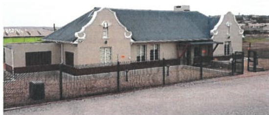
Figure 13: Vredenburg Station Building - Renovated
