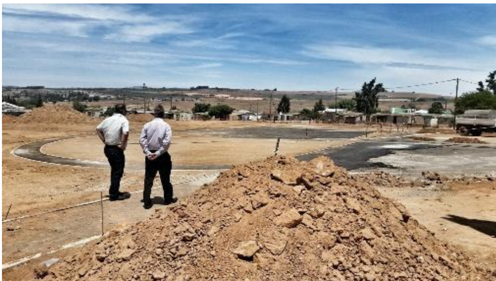
Figure 25: Recreational node currently under construction along Alfa Street in Malmesbury
