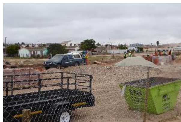
Figure 20: Construction of the Kooitjieskloof Splash Park underway in Vredenburg
