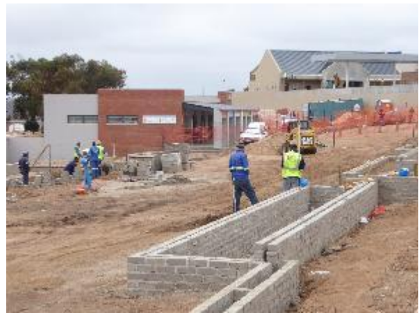
Figure 18: Construction of the Active Box and landscaping underway in Vredenburg
