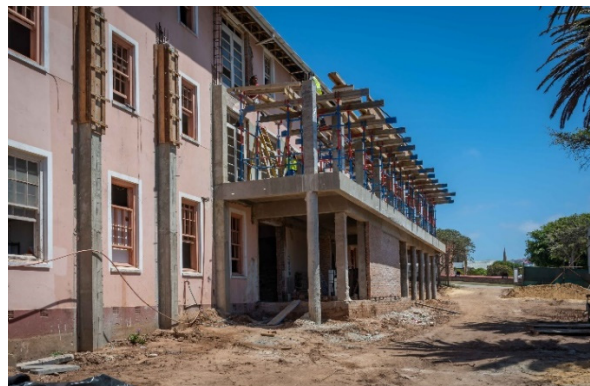
Mossel Bay Shared Services Centre (Mossel Bay Municipality)
