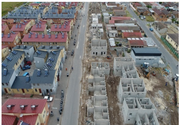
Joe Slovo Housing Project
