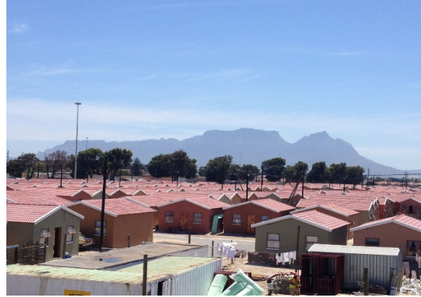
Boystown Housing Project (City of Cape Town)
