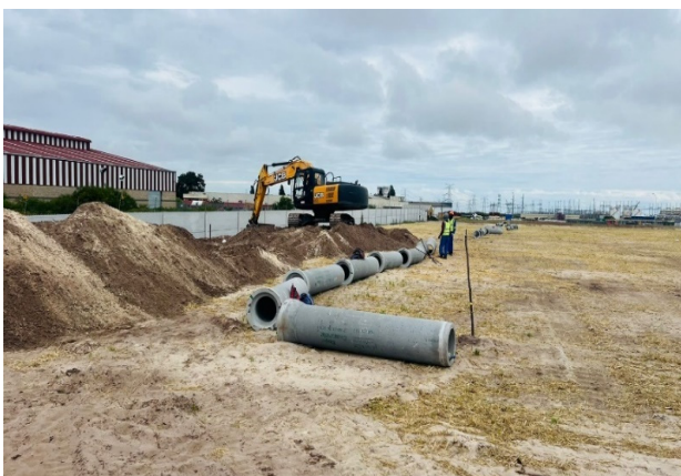
Zone one civils preparation, ASEZ
