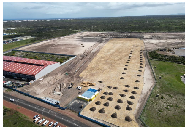
Aerial view of Zone one: Civils work at ASEZ
