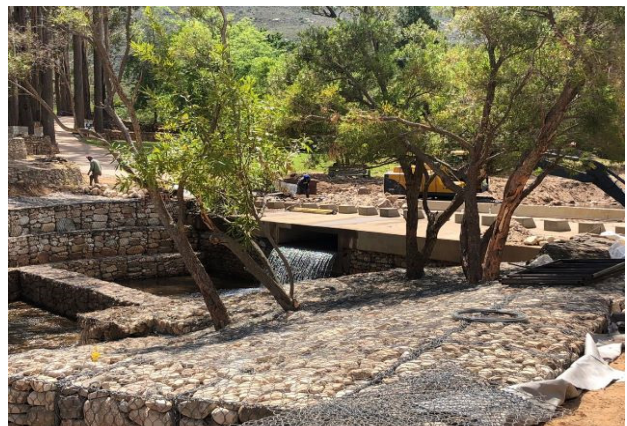
Alegria Low Water Bridge Repairs
