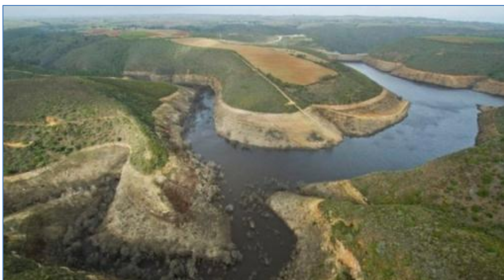
Figure 10.7.2 The Wolwedans Dam
