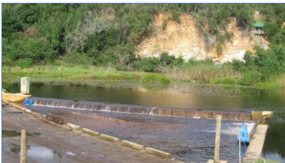
Figure 10.7.4 The Knysna River DWA gauge and Charlesford pumpstation.
