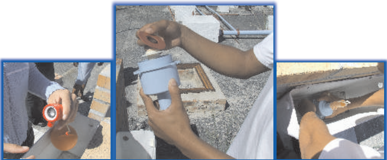
A toilet is retrofitted
