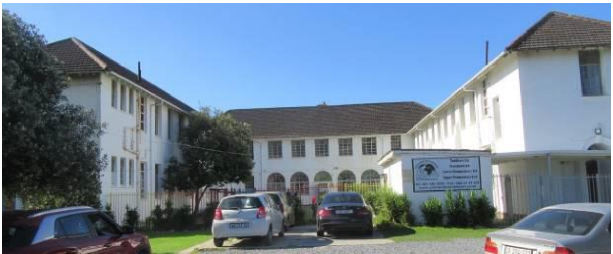
Photograph 4.4: Pinelands Montessori School, Block C.
