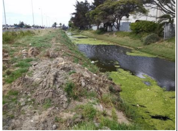
Photo 4: Sediment removal is required at the Bayside canal. Removed sediment should not be stockpiled for periods longer than two weeks.
