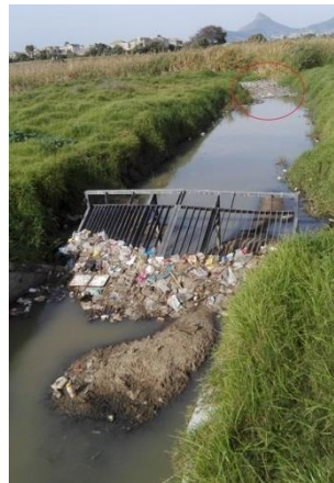
Photo 10: Litter and debris accumulation in a stormwater channel
