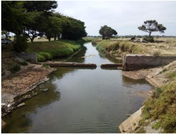
Photo 7: Weirs at the Theo Marais outlet require maintenance
