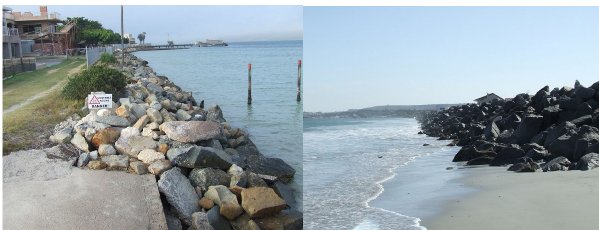
Figure 4-1 Rock revetments along the Langebaan coastline, constructed following storm erosion in 1997.
