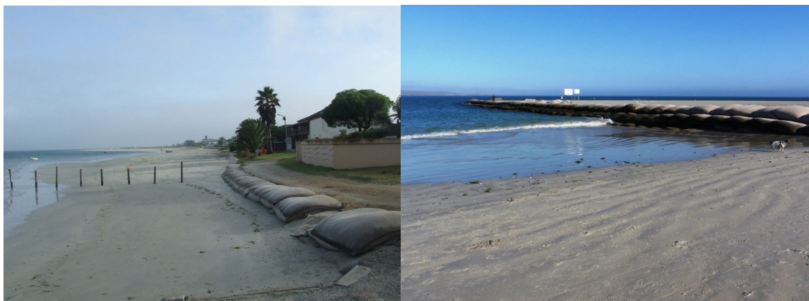
Figure 4-2 Geofabric barriers and groynes along the Langebaan coastline.
