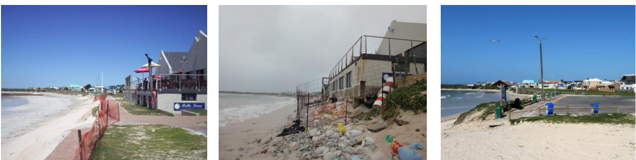
Figure 19: The Nostra Restaurant in Struisbaai progressively undermined by coastal erosion
