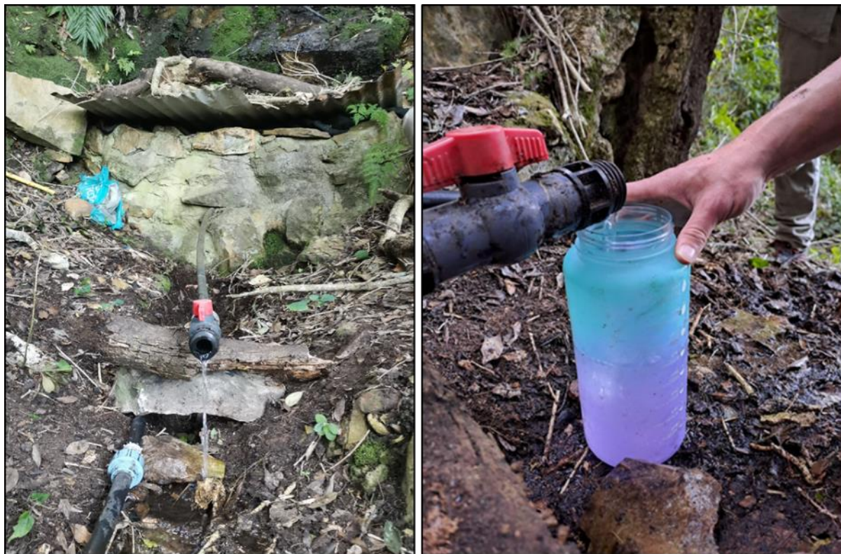
Figure 39: Container fill method tested out in the field at Spring 1.
