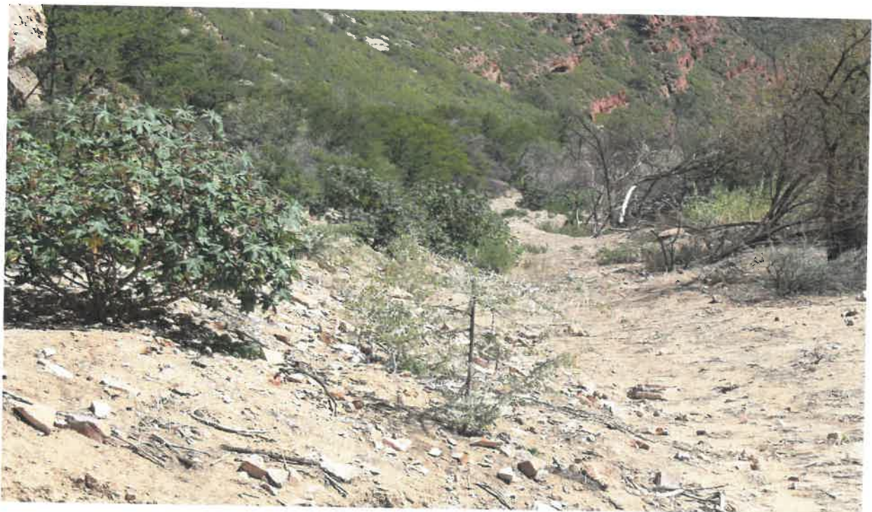
Photo 1: View of the clearing of vegetation and road construction.
