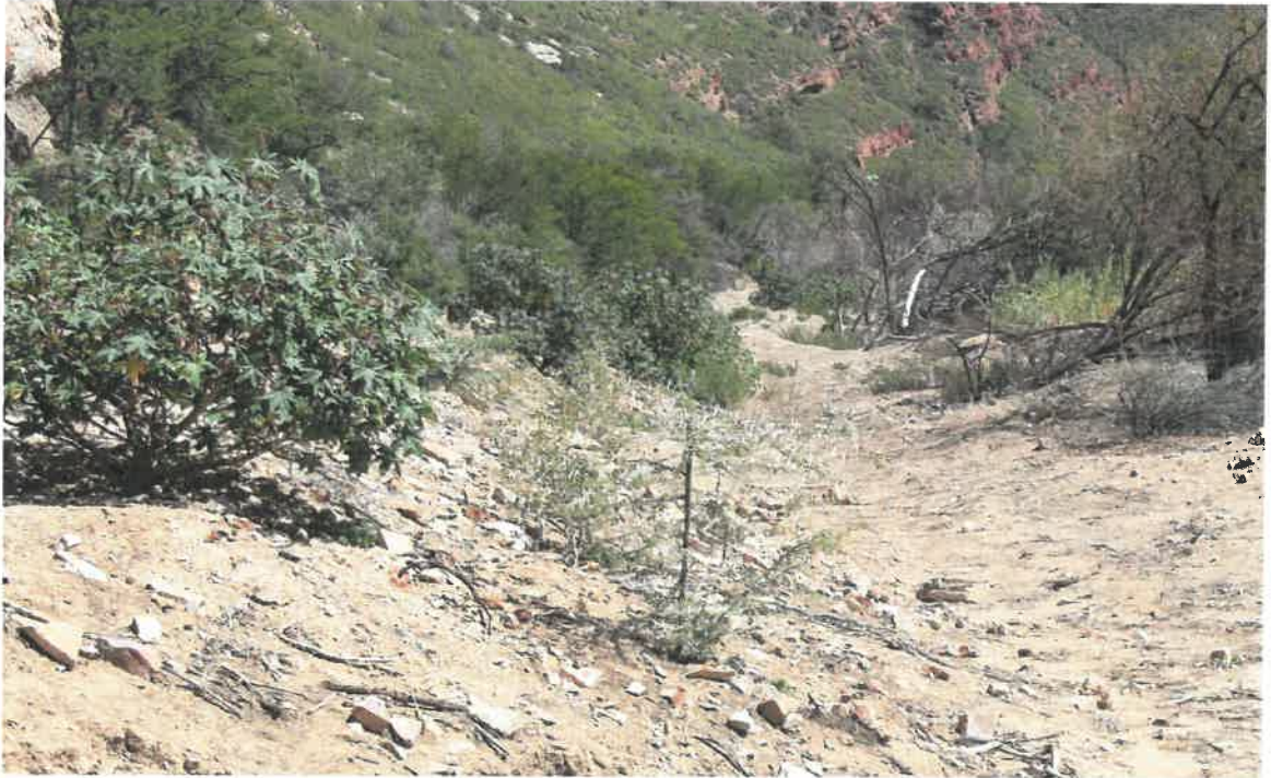
Photo 1: clearing of vegetation and road construction.
