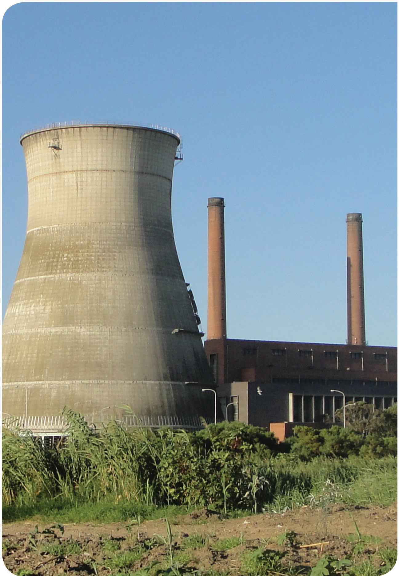
Athlone Power Station and Water Coolers. Wikimedia Commons - Free media repository.
