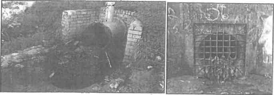
Figure 20: Example of litter traps from stormwater outlets.
