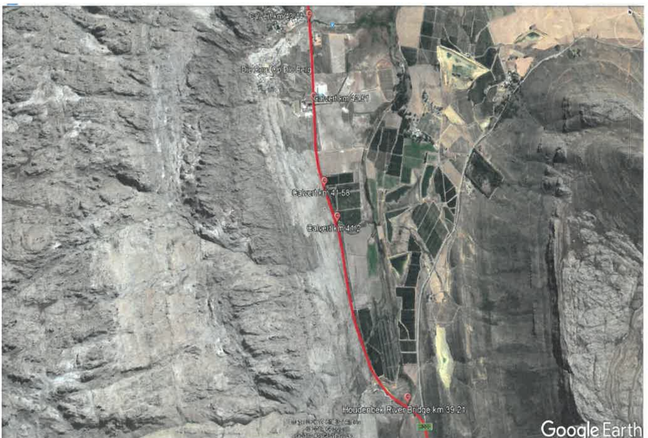
Figure 2: Depicting the 4 culverts and the Houdenbek River Bridge, proposed to be upgraded.
