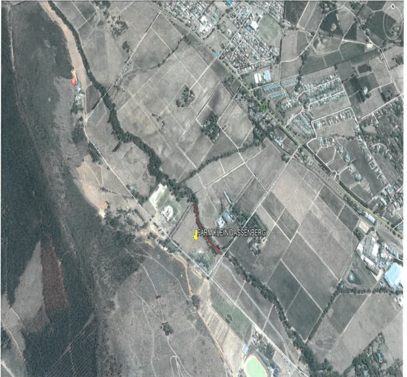
Figure 1: Locality map of the gabion revetments on Farm Klein Dassenberg No. 1551, Franschoek.
