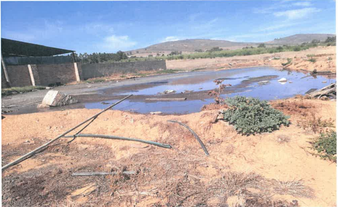
Photo 3: Unlined effluent pond
