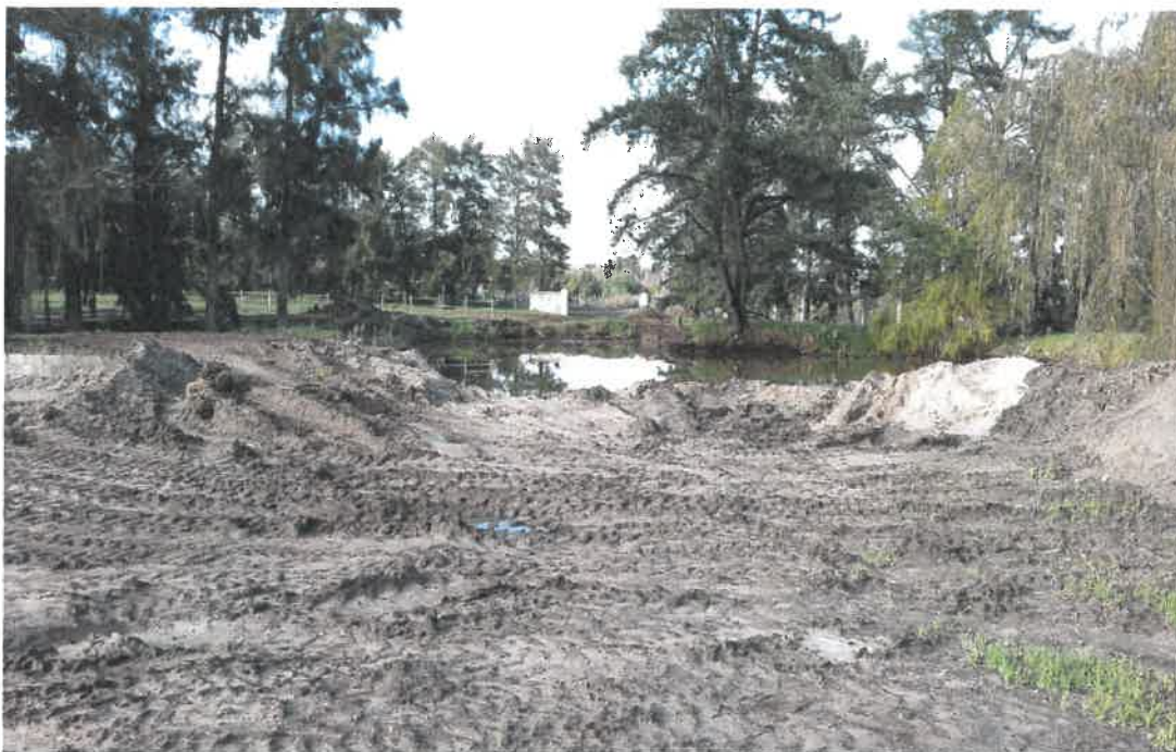
Photo 1: Removal of soil from the in-stream dam.
