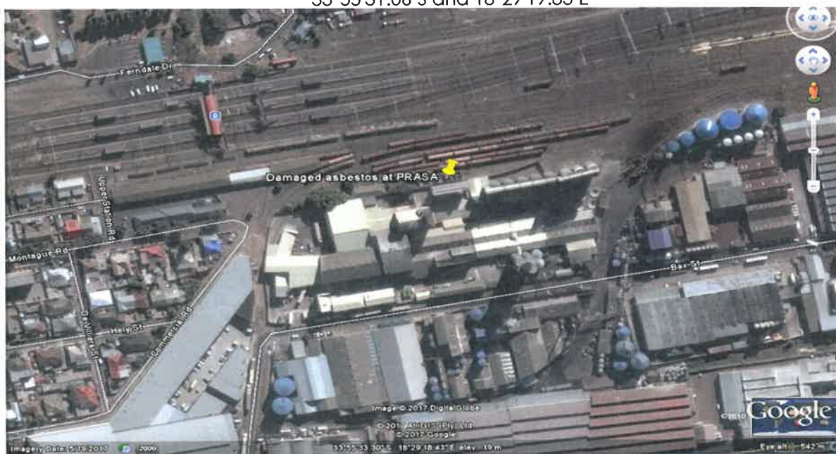
Aerial Map: Location of illegal storage of hazardous waste (asbestos) at PRASA's old building.
