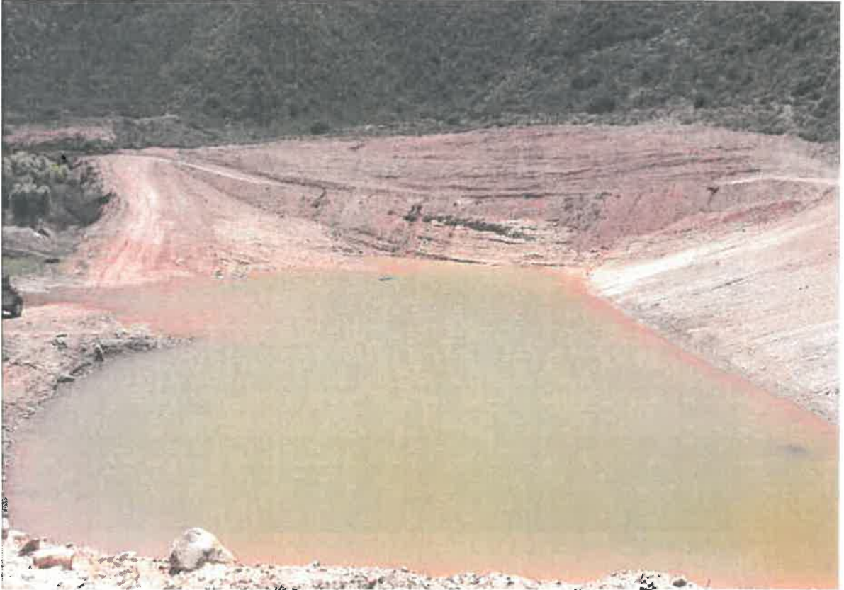
Photo 1: A view from inside the expanded dam.
