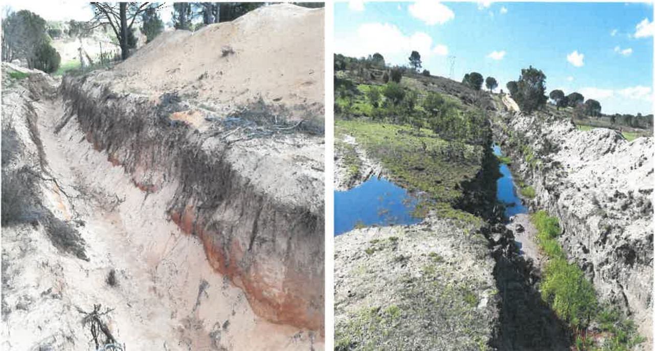
Photo 3-4: Moving of soil and sand from a watercourse
