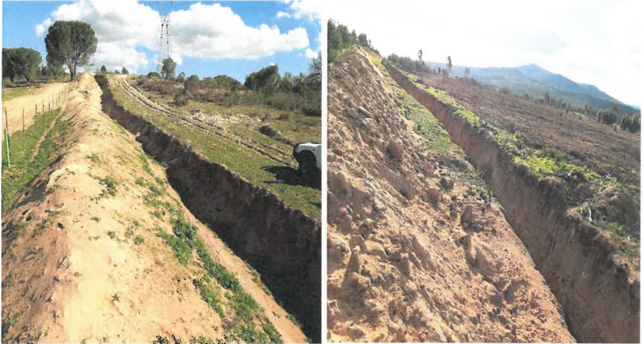
Photo 1-2: Clearing of indigenous vegetation and construction activities
