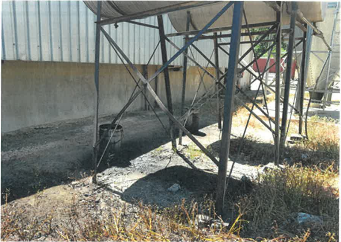
Photo 8: Unbounded fuel/oil storage tanks and spill of oil on the ground on the property.
