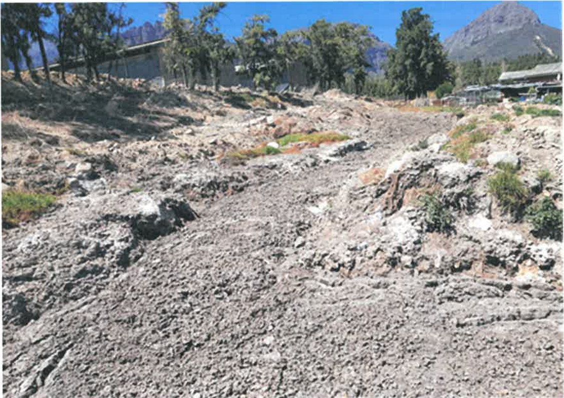
Photo 6: A trench of chicken manure emanating from the facility close to residents on the farm
