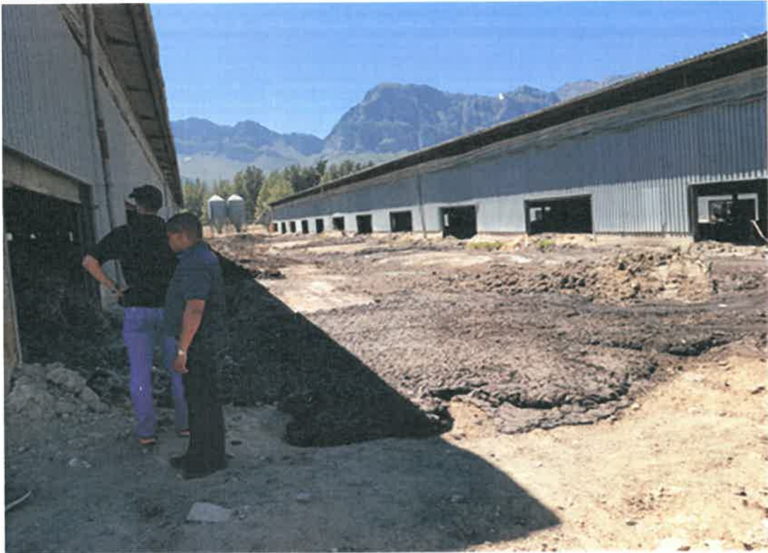
Photo 2: Seepage of wet chicken manure from the chicken houses.
