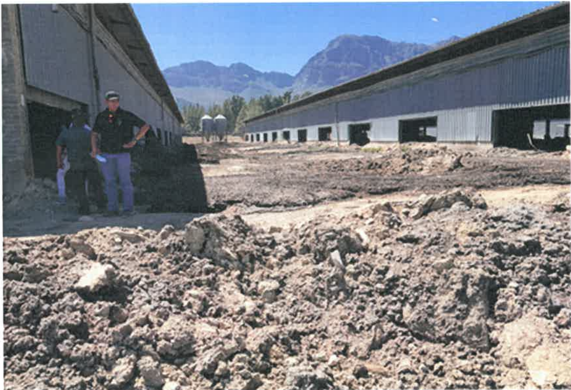
Photo 3: Wet and dry chicken manure stored directly on the ground and flowing into adjacent trenches.
