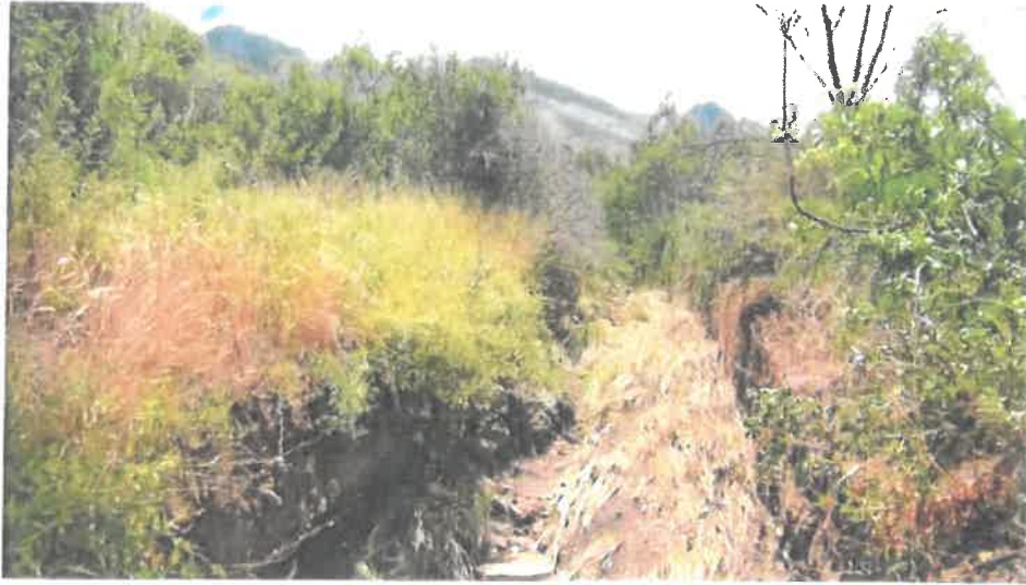
Photo 2: View of the channel that was constructed to divert the water away from the Efflux Cave opening.
