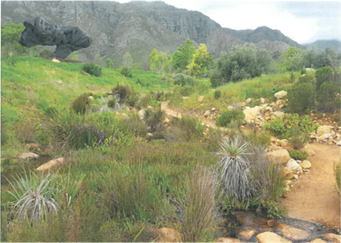
Photo 1: Construction of a walkway and sculpture display within a watercourse.
