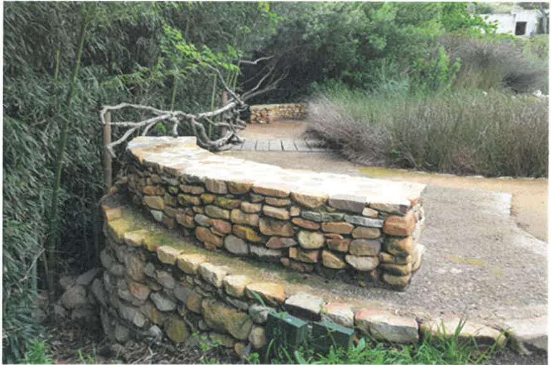
Photo 5: Concrete weir built within a watercourse.
