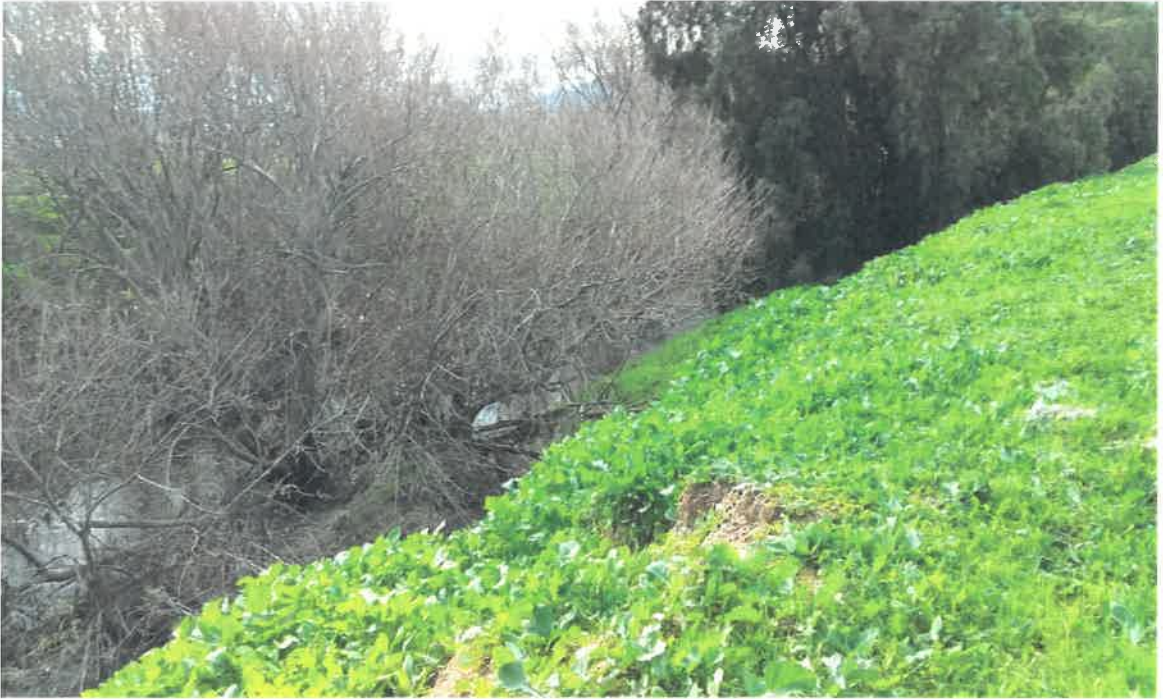
Photo 1: View of infilling within the Eerste River and raising of its banks.
