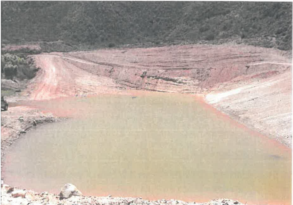
Photo 1: A view from inside the expanded dam.
