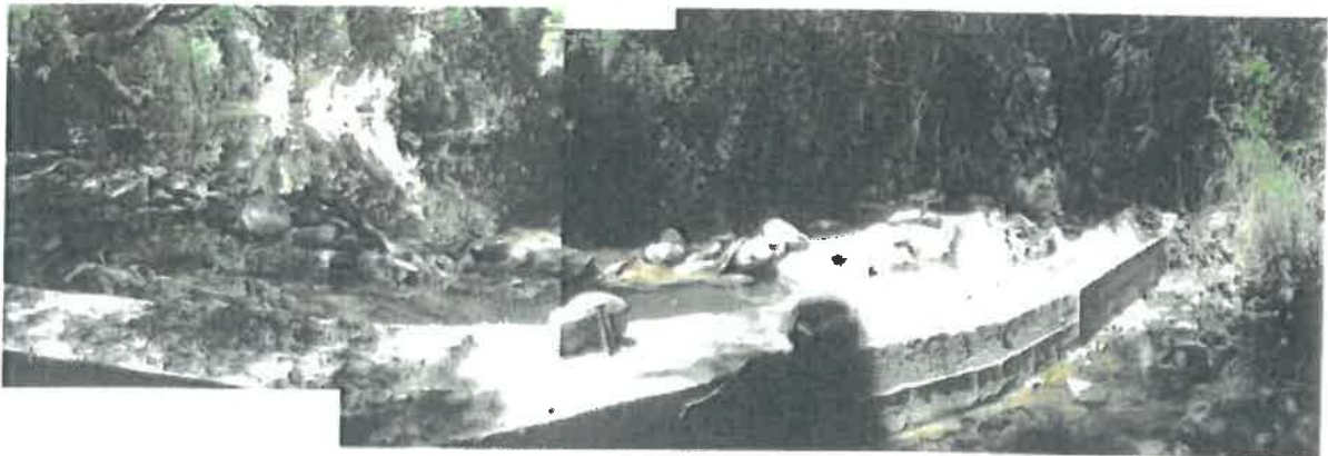
Photo 1: Development of a weir with the watercourse (Nels Rivier, Calitzdorp).
