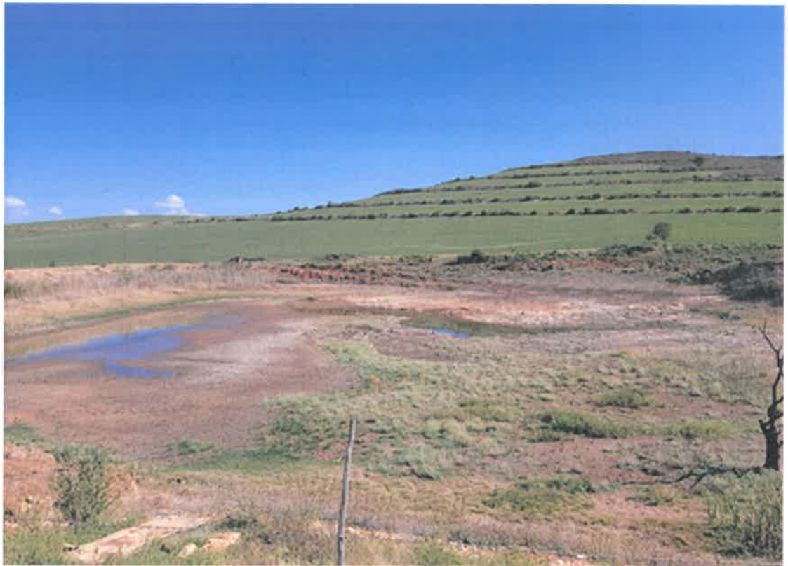
Photo 1: The extent of the dam as viewed from the eastern direction.
