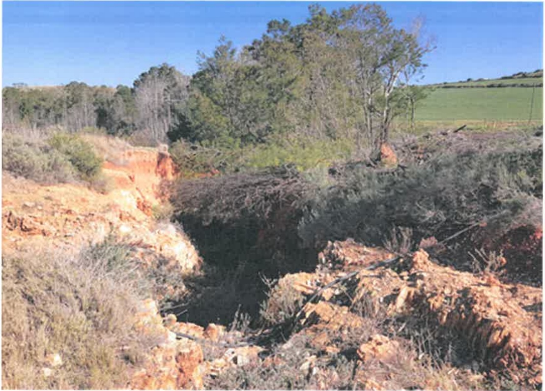
Photo 4: The dam overflow/spillway.
