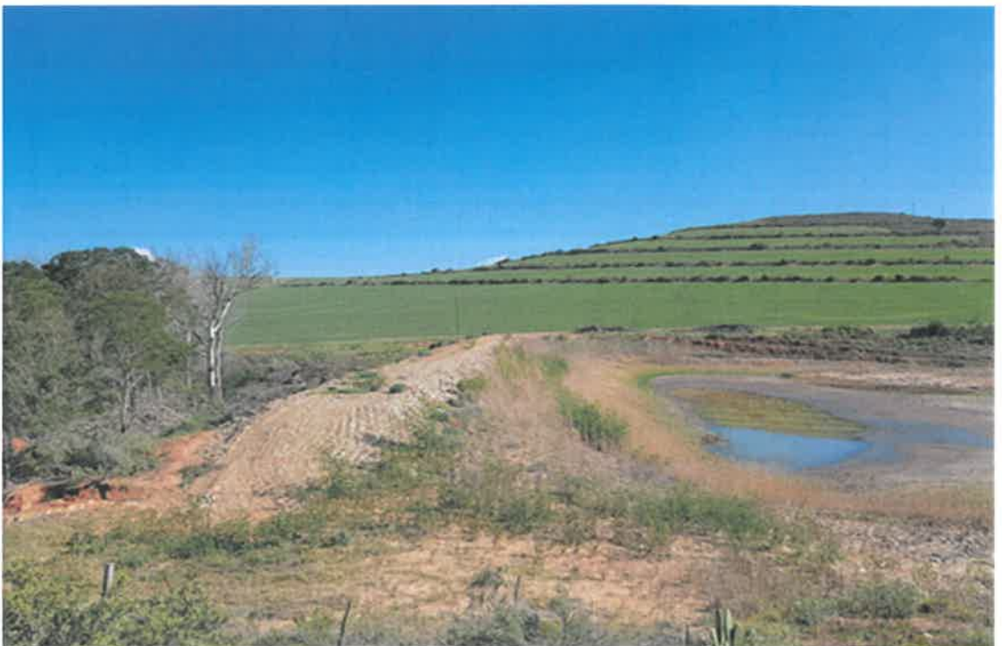
Photo 3: The dam wall which was repaired.
