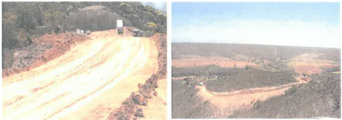
Photo 4: Construction of a road more than 4m wide
