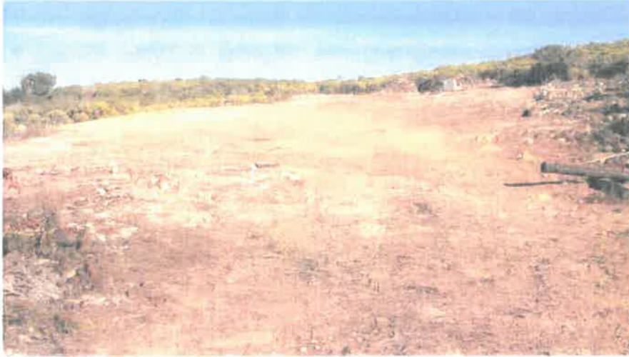
Photo 3: Clearance of vegetation
