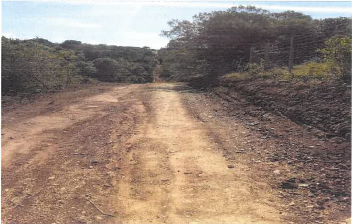
Photo3: Constructed main road
