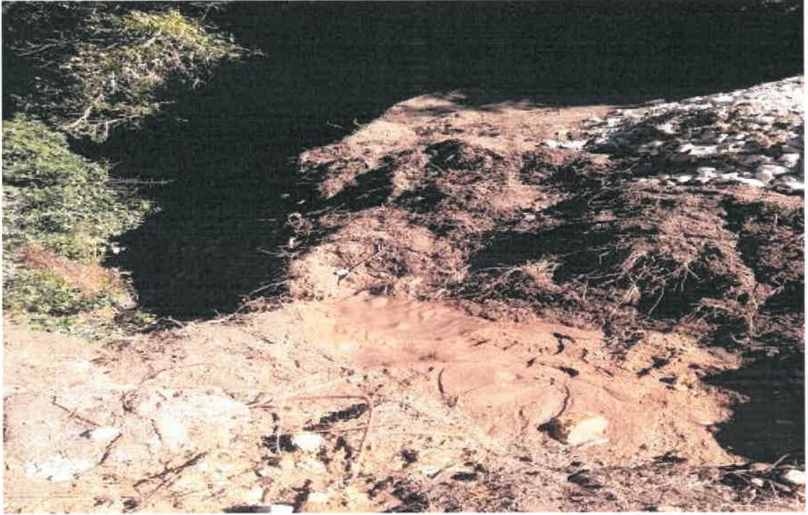
Photo4: Infilling in the river crossing
