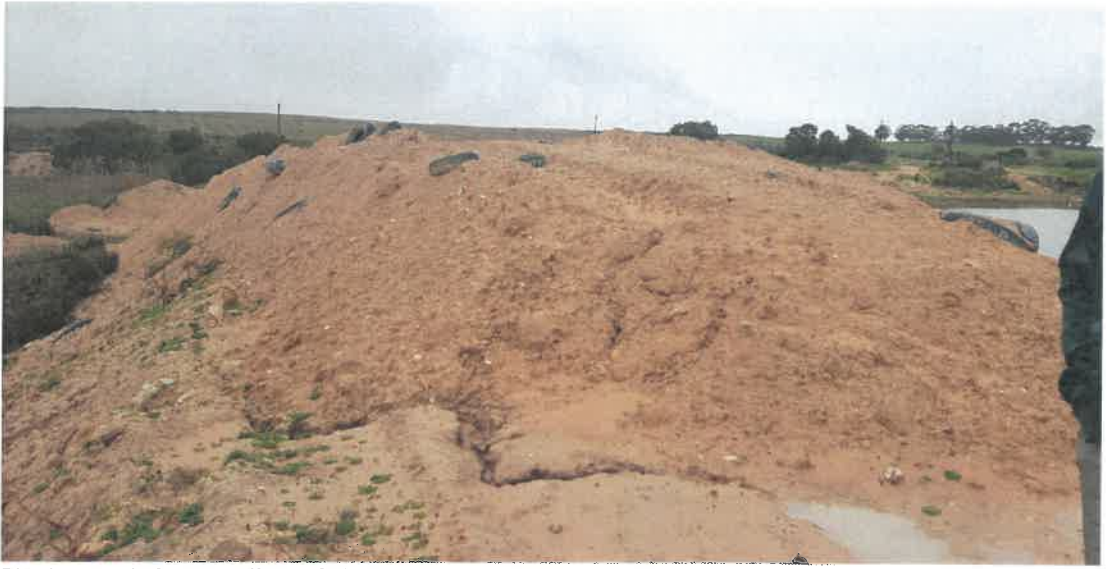
Photograph 1: A portion of dam-wall comprising of clay and tyres
