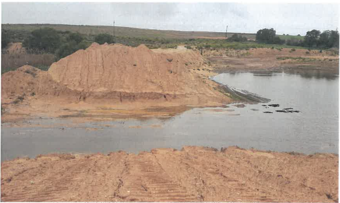
Photograph 2: Area where in-stream dam-wall was removed.
