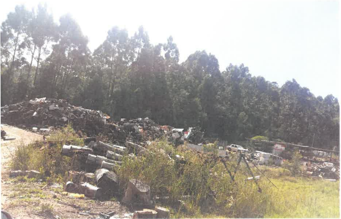
Photo4: Close view of the illegal storage of waste at De Kop Quarry erf 16/422, Harkeville
