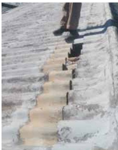
Figure 1: Access gained by removing some of the roof tiles.
