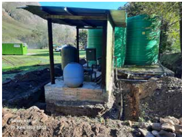
Upgrading of the borehole system and replacement of ageing water storage tanks.
