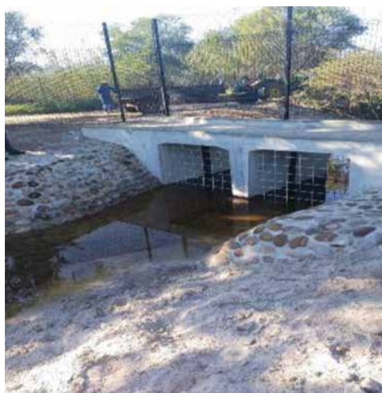
Installation of security fence and remedial work done to the bridge at GD facility.
