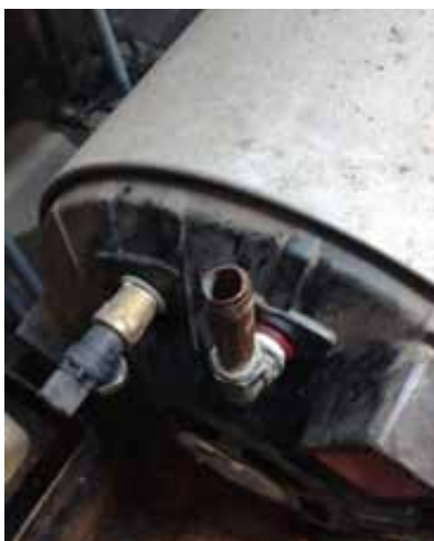
Figure 2: Removal of copper pipes to the geyser.
