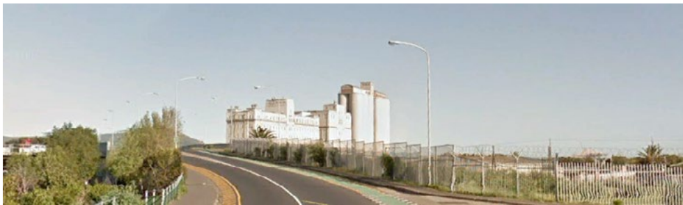
Figure 4.10. Transnet site north of the study area
