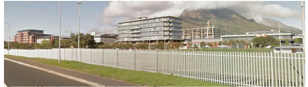
Figure 4.13. View of Malta Park towards Observatory
