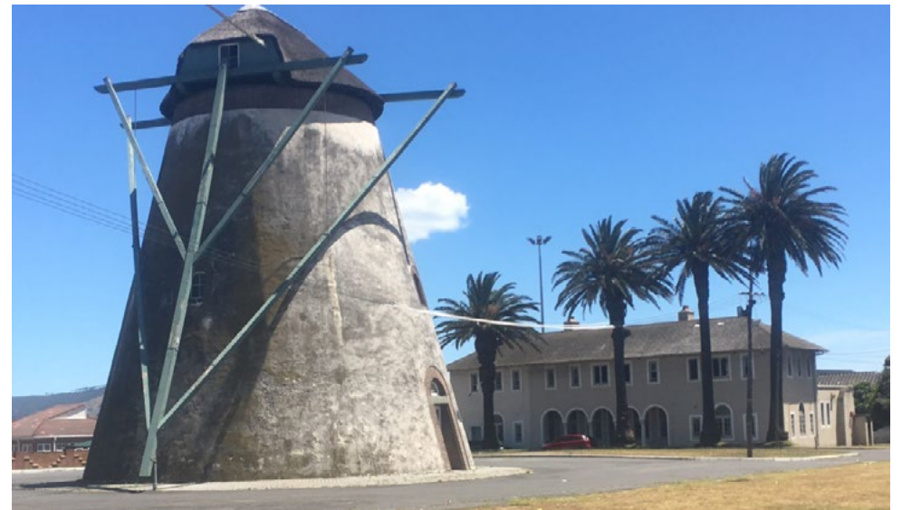
Figure 4.19. Old admin building and Nieuwe Molen at Alexandra Hospital.
