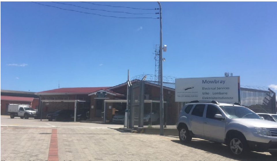
Figure 4.21. City of Cape Town utilities building in Ndabeni Triangle
