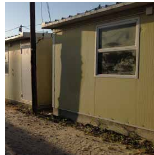
TRUs are in a fenced-off area with security.
