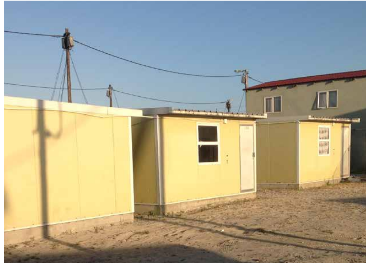
Each unit has a working power supply box.
