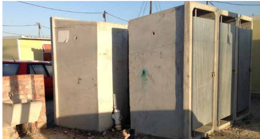
TRA 6 has stand alone toilets and taps with sinks.
